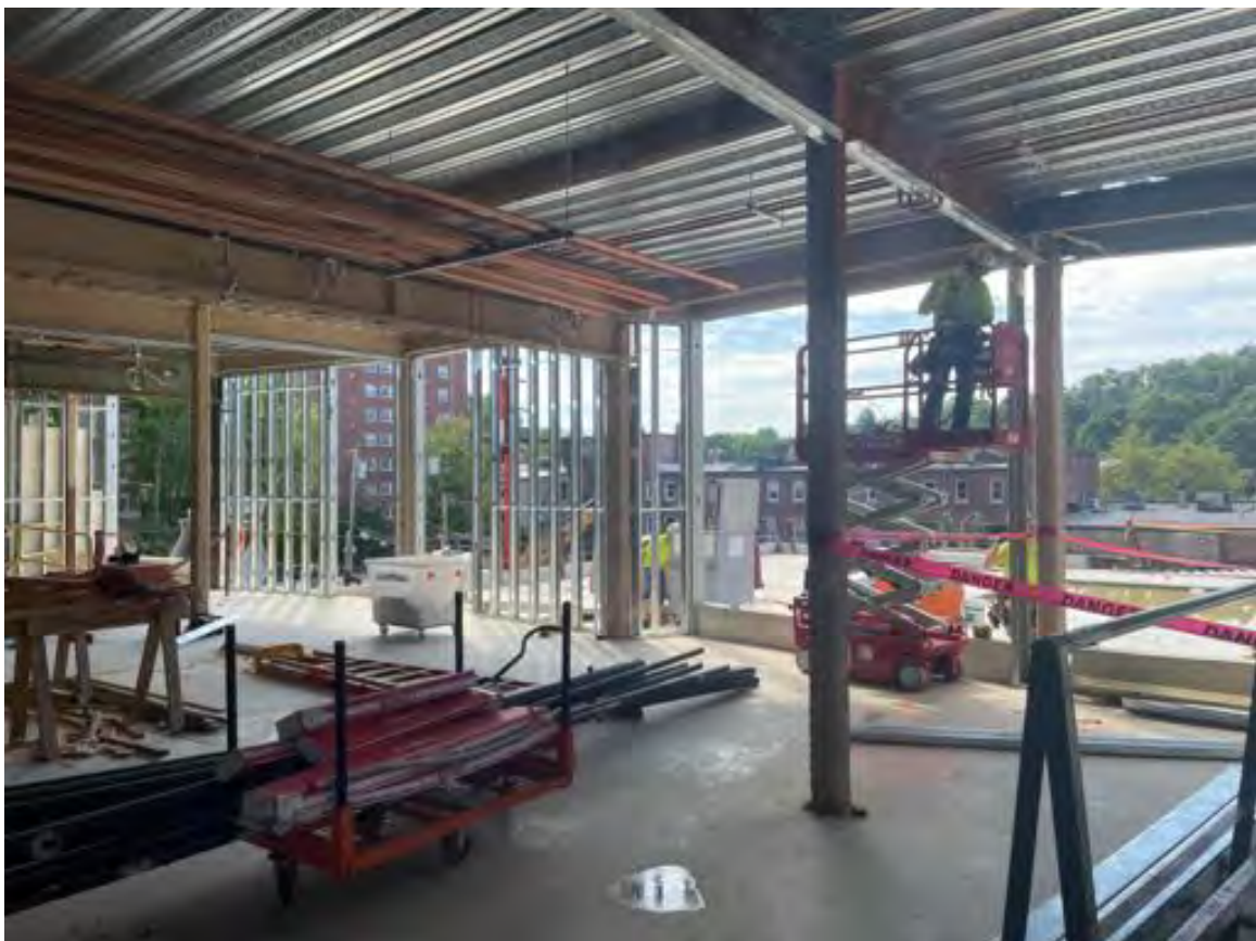
Level 2 exterior framing.
