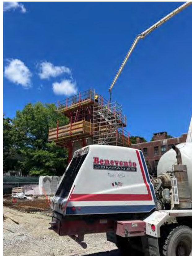
Concrete pour, 3 rd lift Core B.
