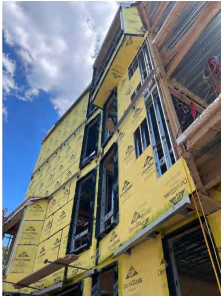
Waterproofing, West elevation Area C.
