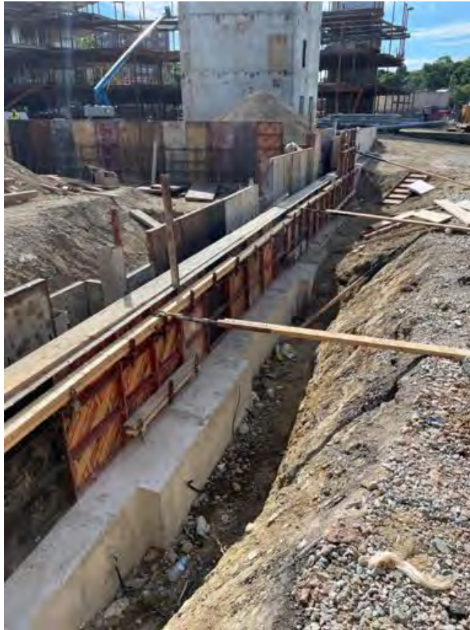
Forms and rebar, line BD-Core B foundation wall.
