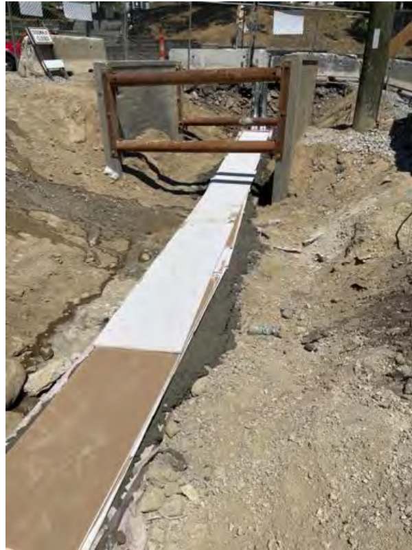
Ductbank capped with concrete.
