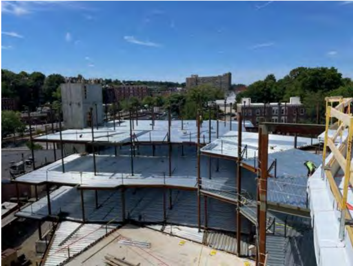
Metal deck, level 4.
