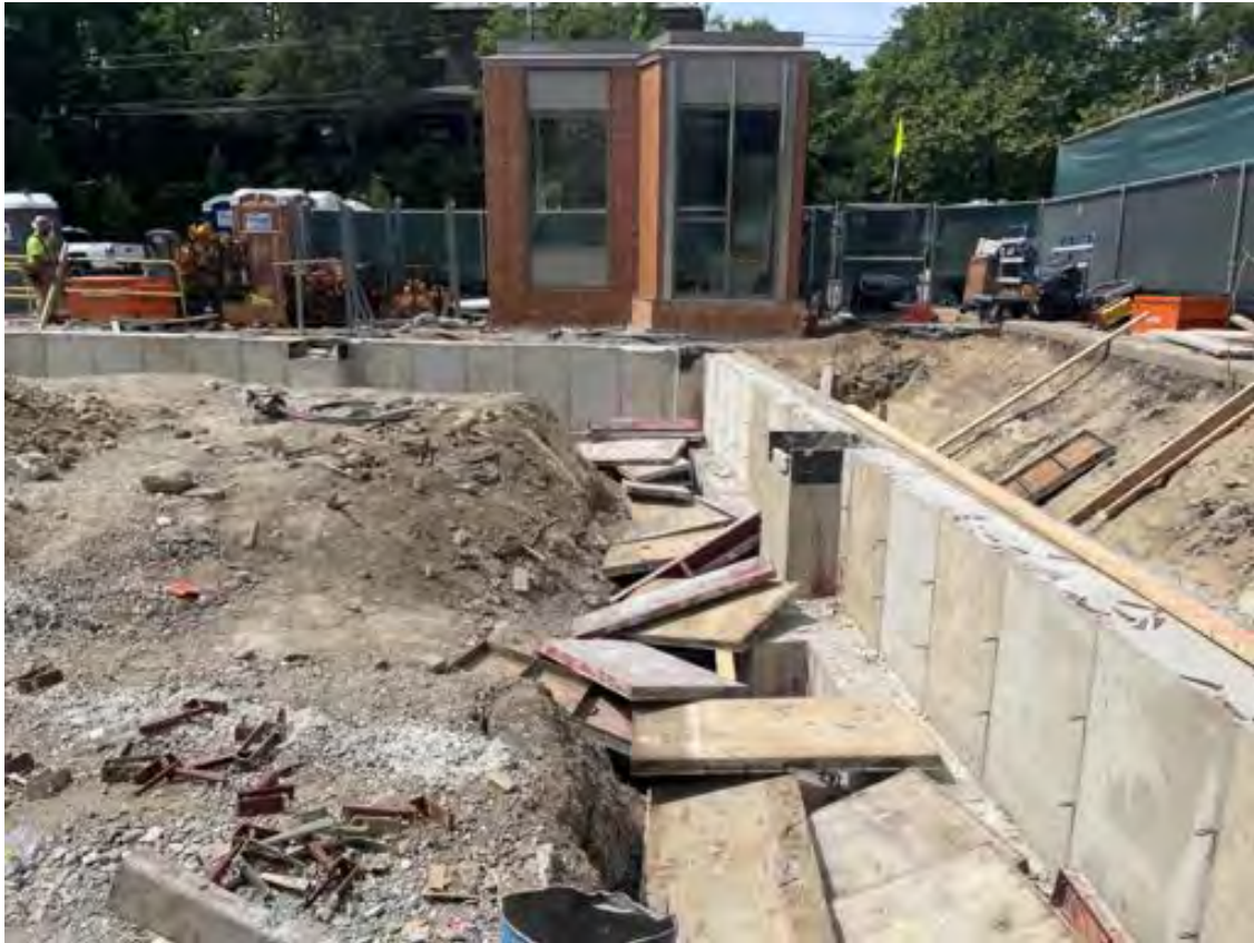
Foundation walls stripped, Area B.
