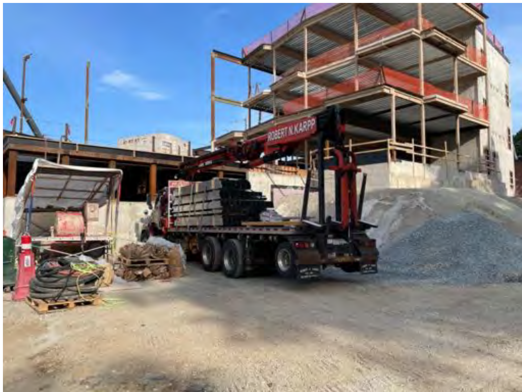
Delivery of metal studs.
