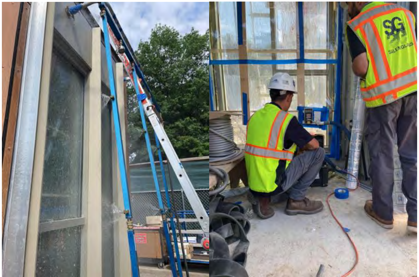
Window performance tests @ mock-up. (Windows passed)
