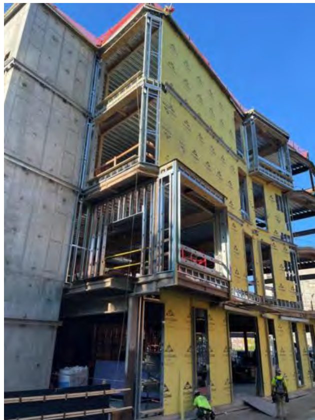
Blocking ongoing at West elevation, Area C.
