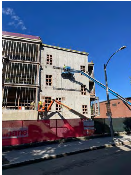
Brick shelves, North elevation Area C.
