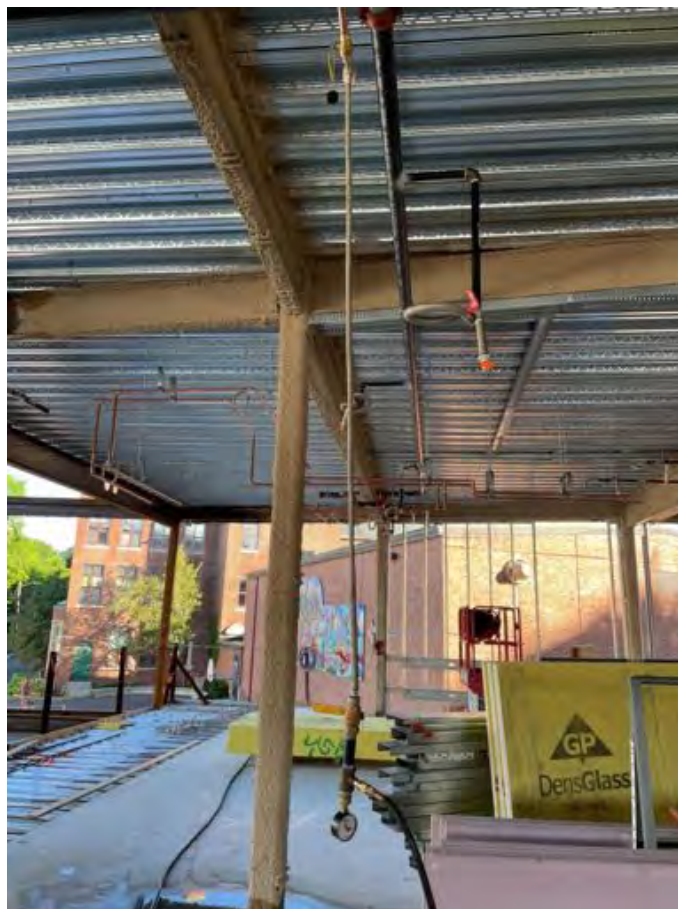
Pressure testing plumbing, level 3 Area C.
