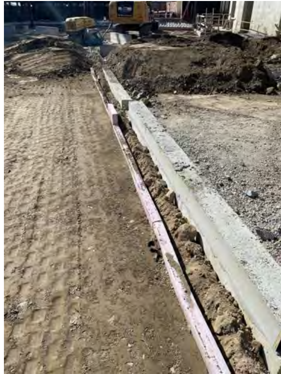
Insulation at line BQ completed.
