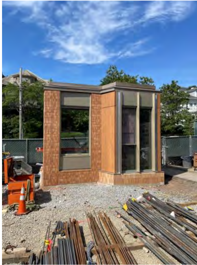
Current state of mock-up.
