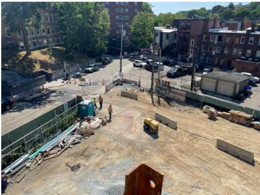
Water main chlorinated and flushed. Pressure test passed.
