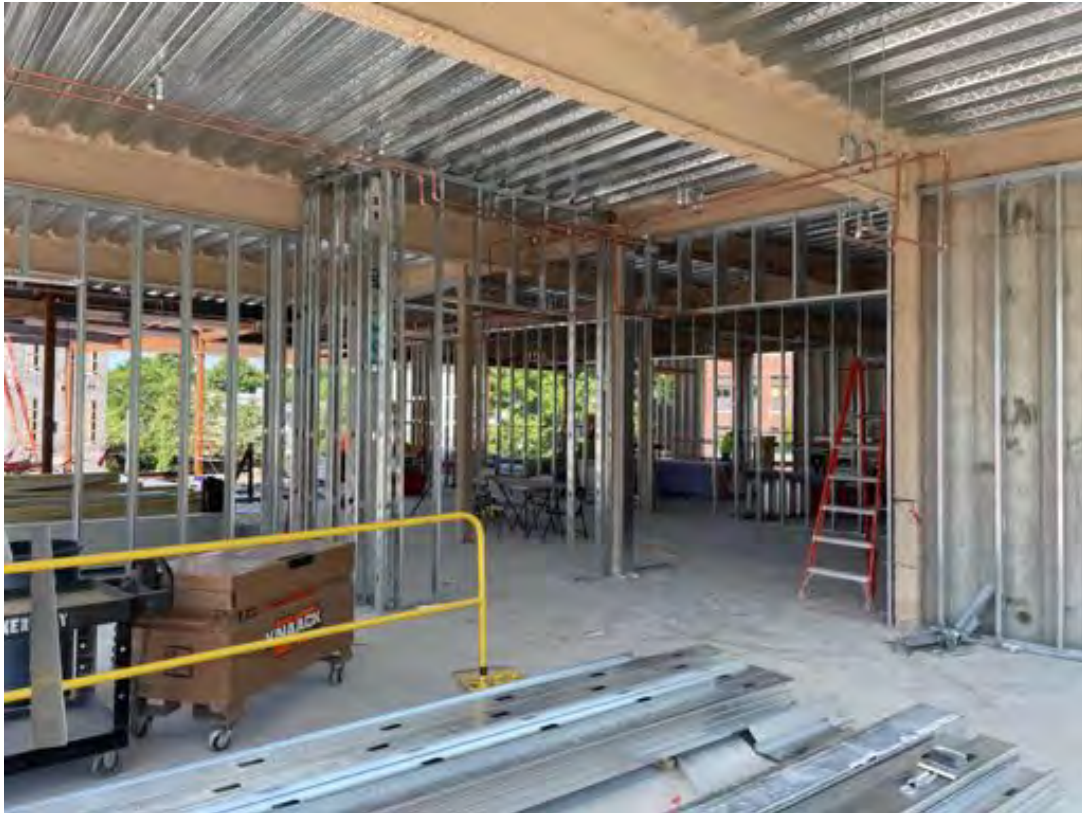
Interior framing level 3, Area C.
