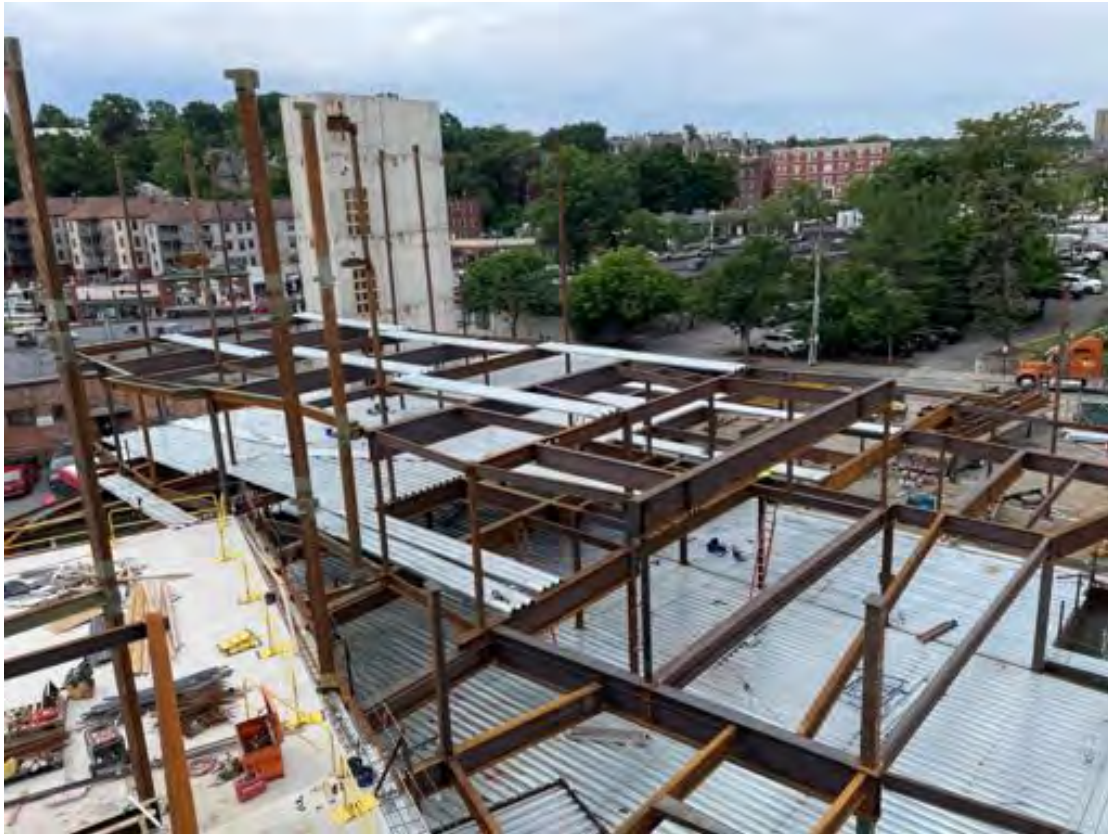
Current status of steel, Area A.
