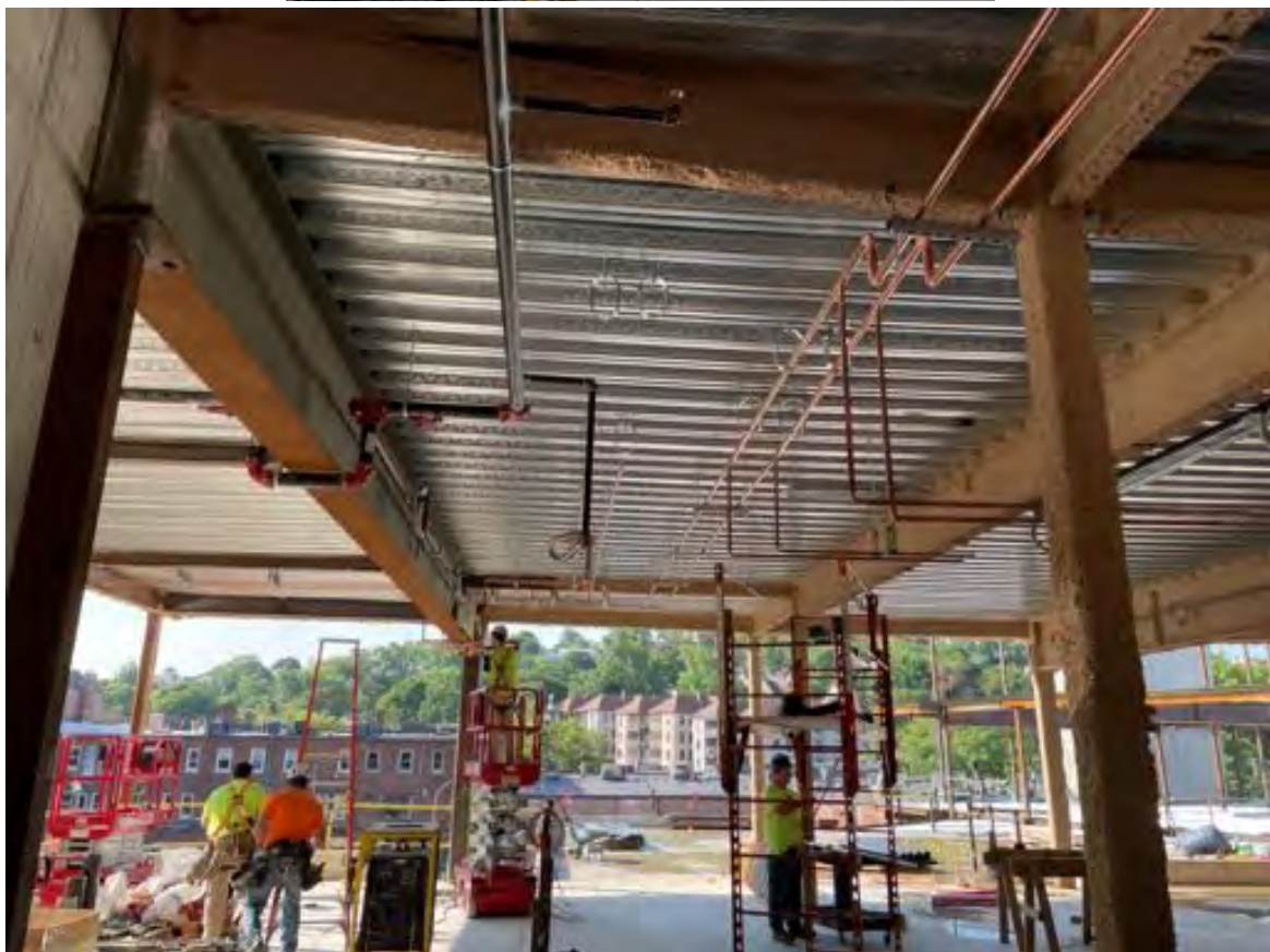
MEP progress, 2 nd floor.
