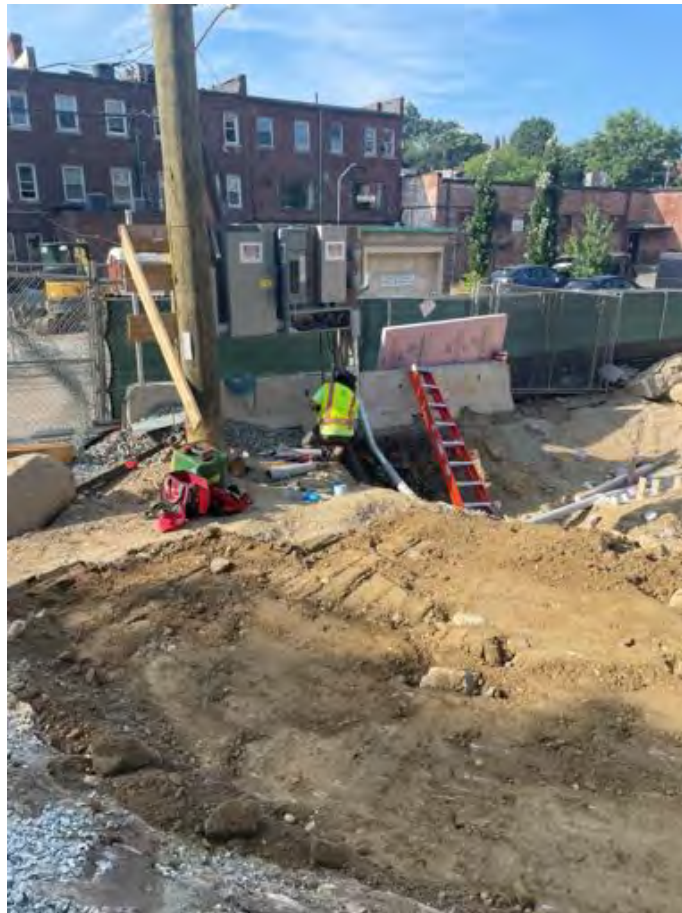
Installing temporary electrical service.
