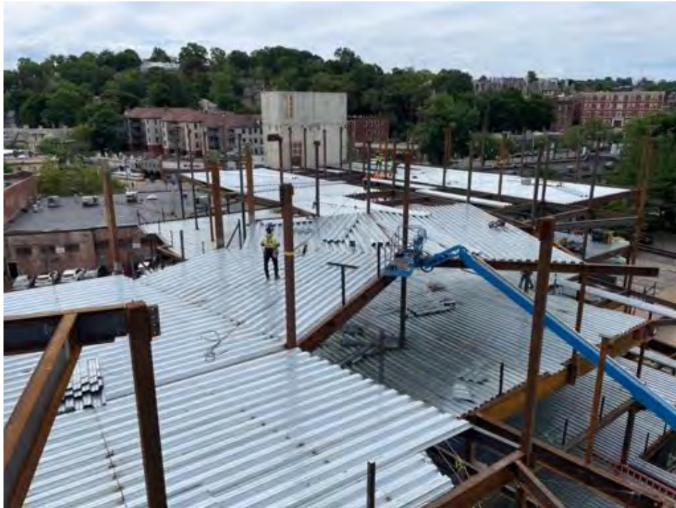
Metal deck, level 4 Area A.
