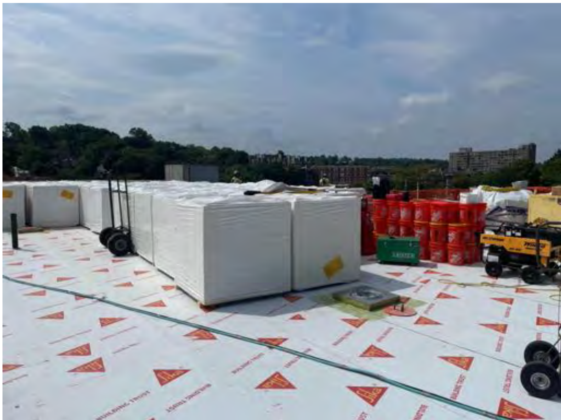
Roofing materials, Area C.
