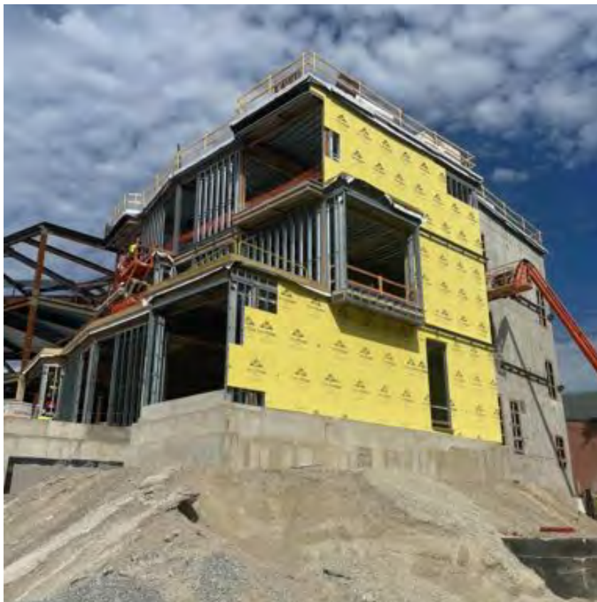
Exterior sheathing/framing progress, NE elevations Area C.
