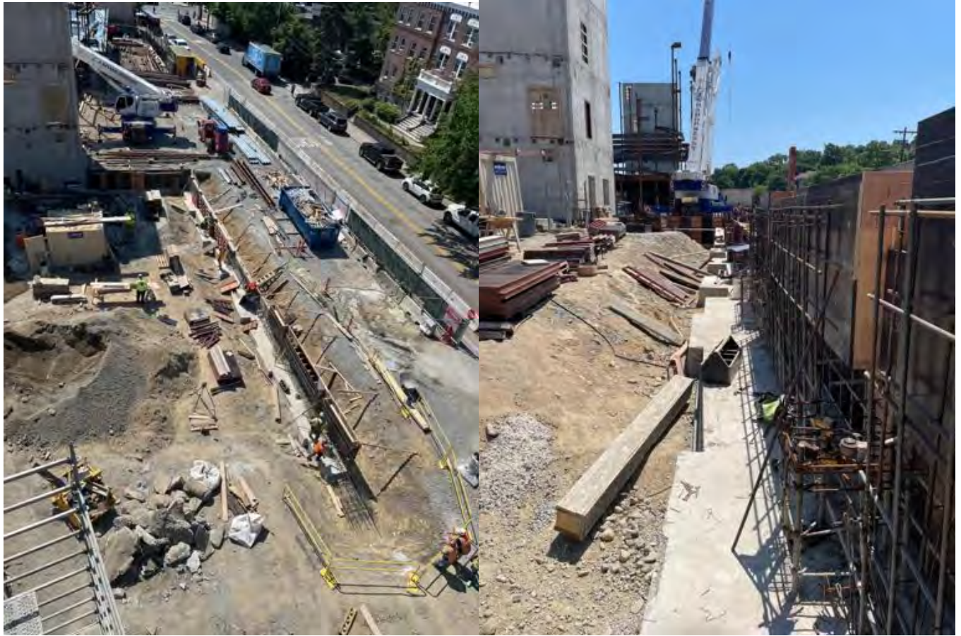
Footings/foundation forms at line BD.
