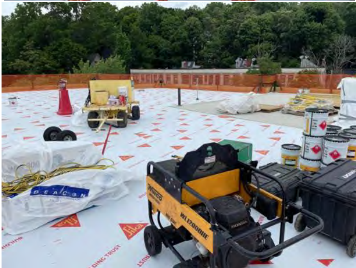
Roofers mobilized and started at Area C.
