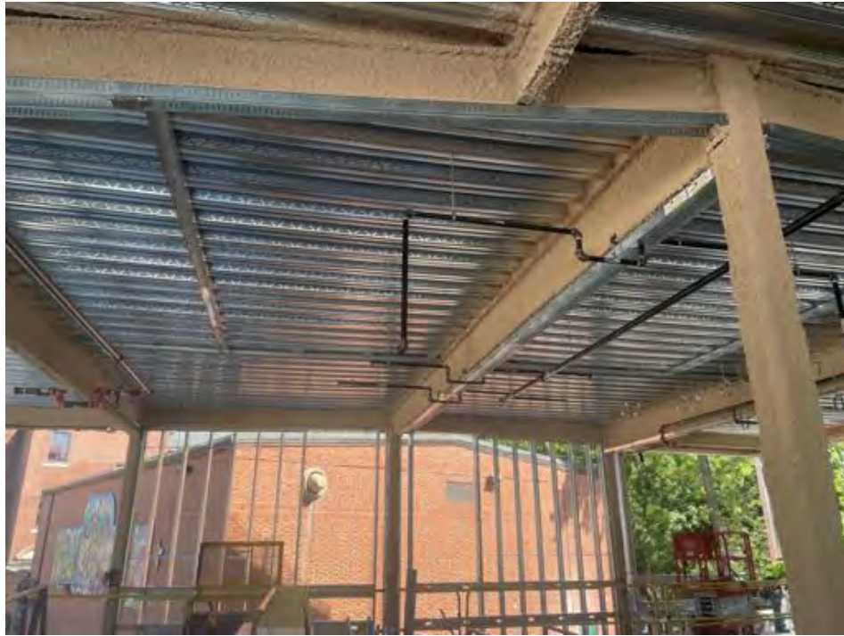
Hangers, strut and pipe being installed, Area C.
