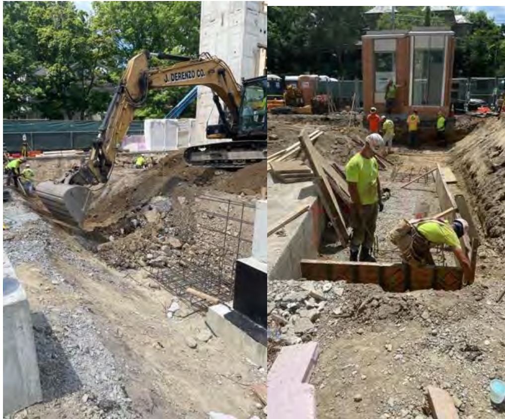
Excavation, forms and rebar for footings, Area B.
