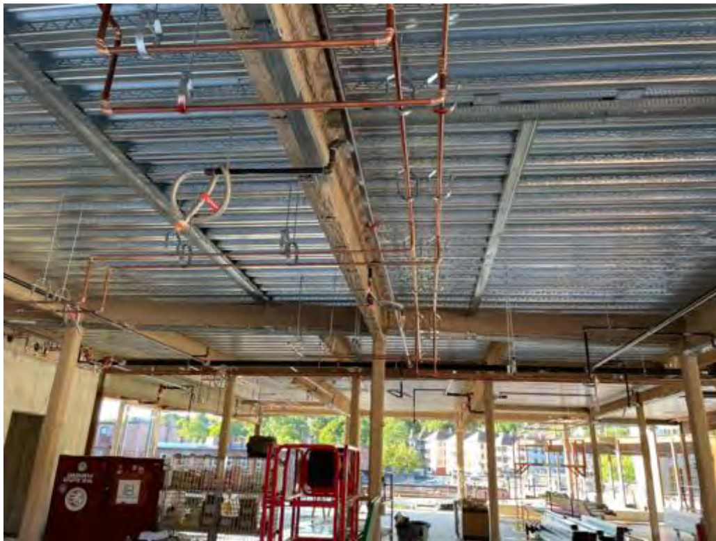
MEP piping ongoing, level 2 Area C.
