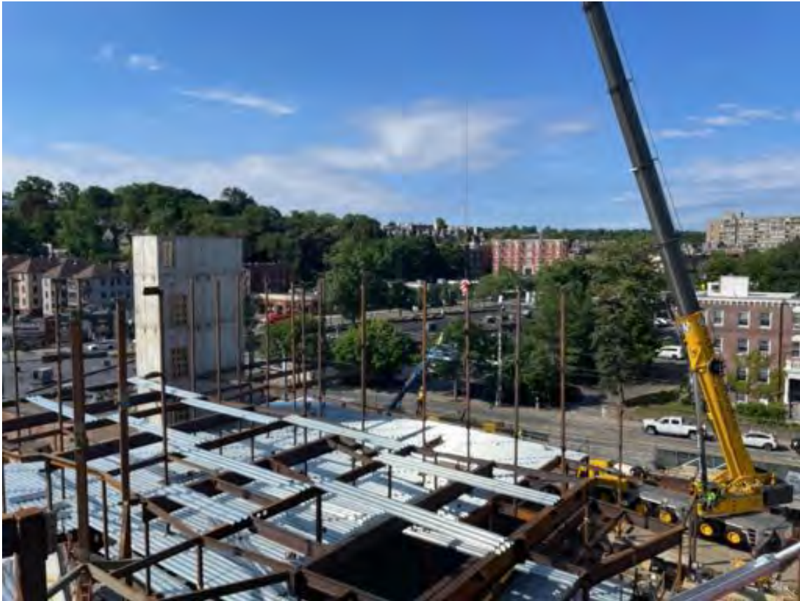
Steel erection ongoing.
