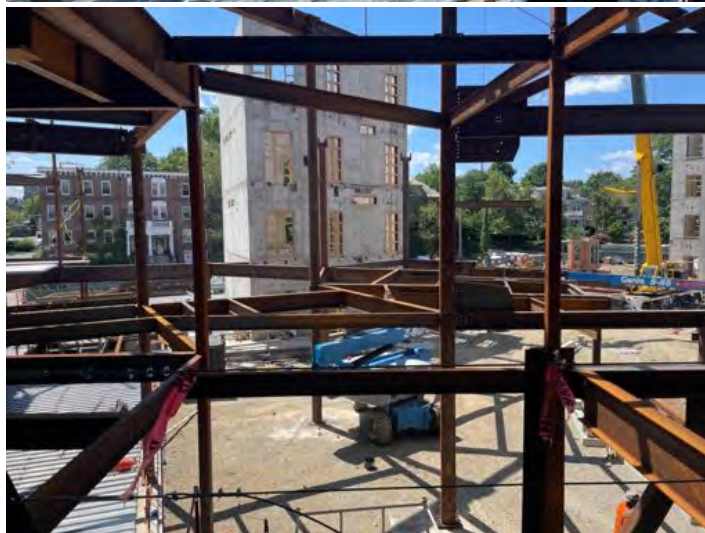
Steel erection, Area A/B/C.
