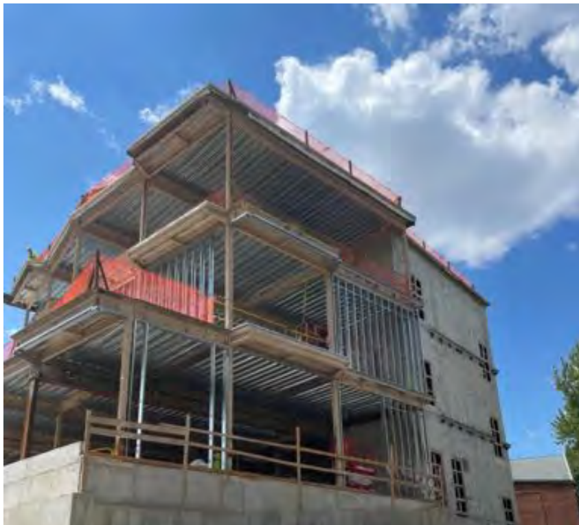
Exterior framing, North and East sides.
