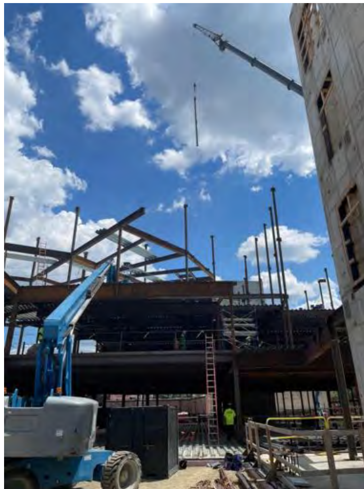
Steel erection, Area A 4 th floor.
