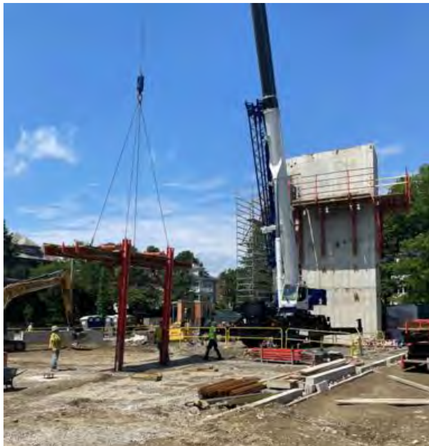
Core B forms being removed.
