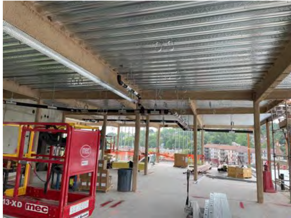
Mech pipe hangers, Level 4 Area C.
