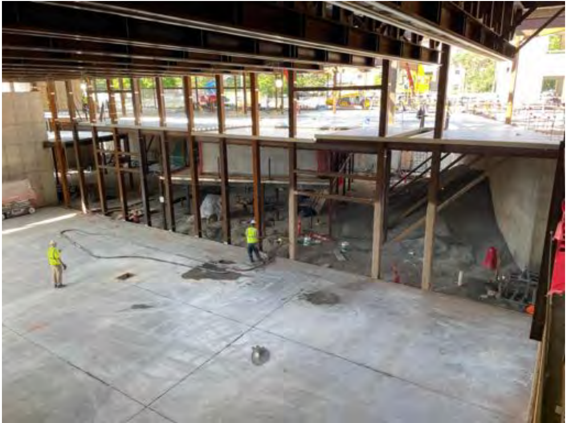
Spray-on fireproofing, basement level.
