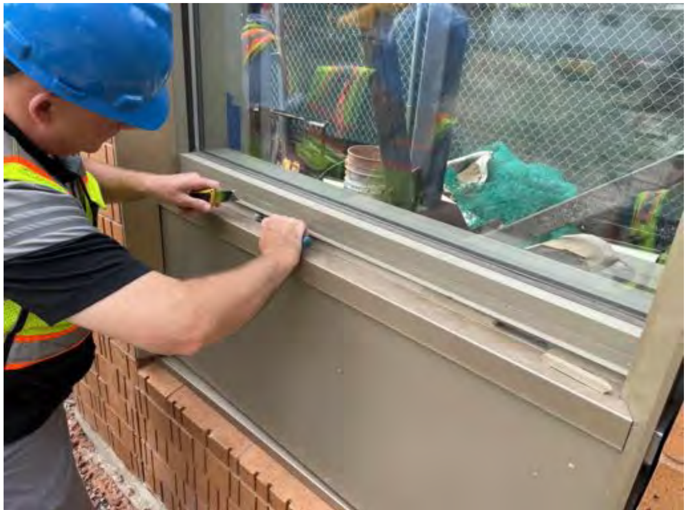
Caulking pull test @ mock-up.
