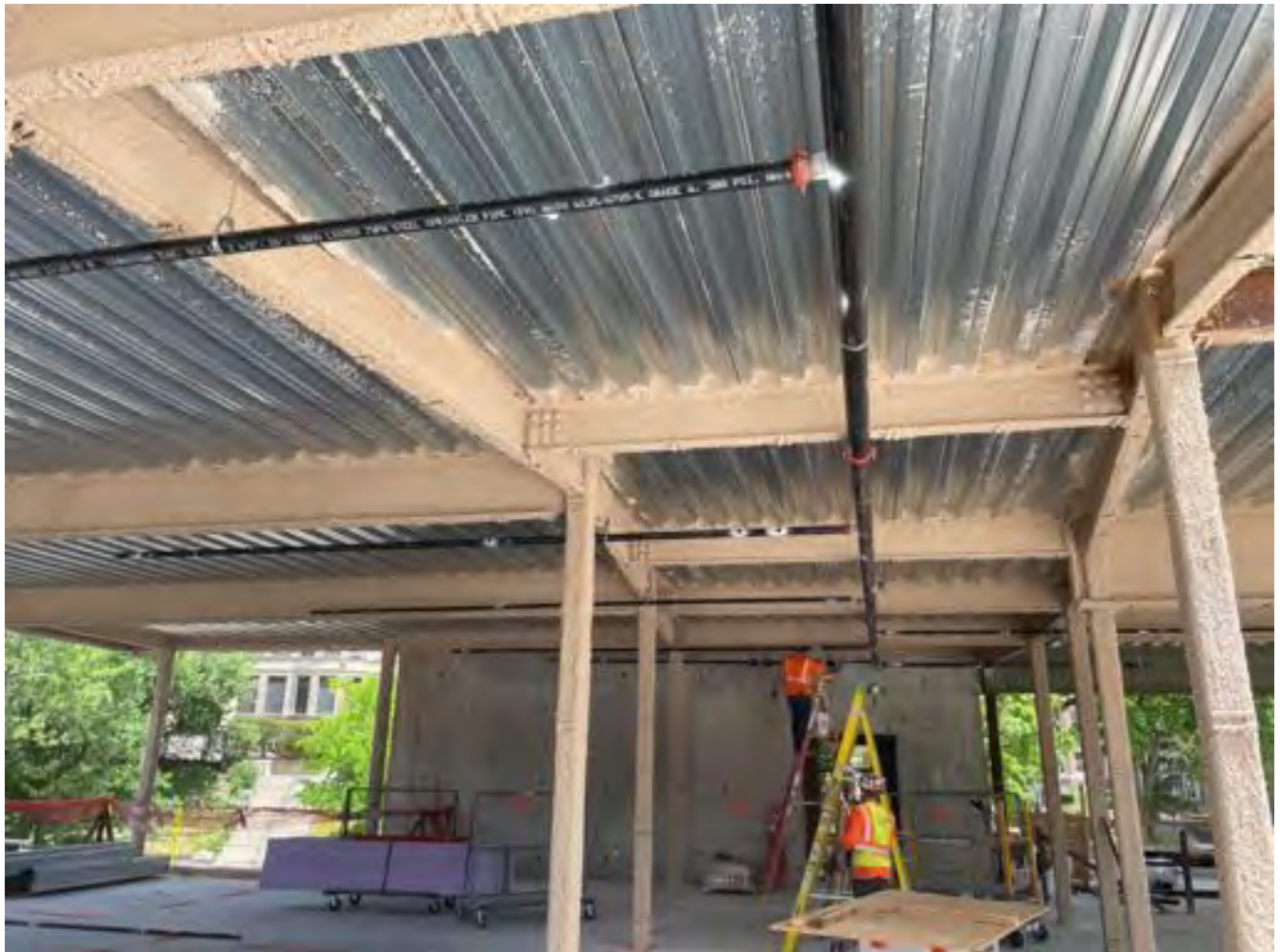
Installing sprinkler pipe, Level 2 Area C.
