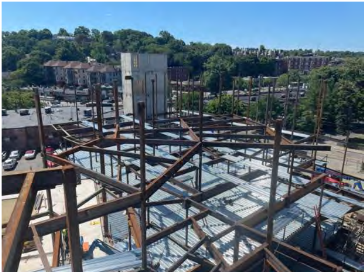
Steel erection, Area A ongoing.
