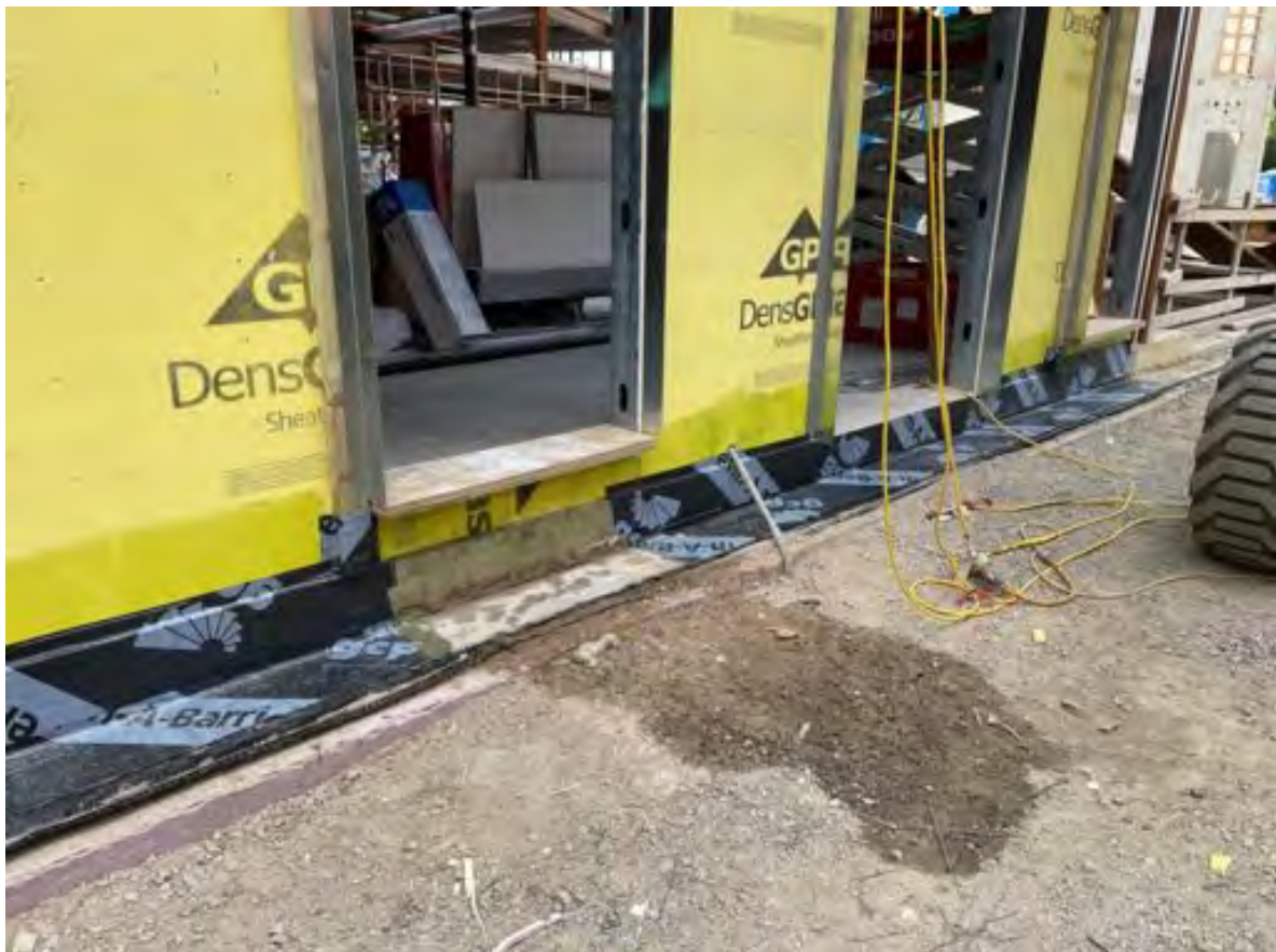
Waterproofing, West elevation Area C.
