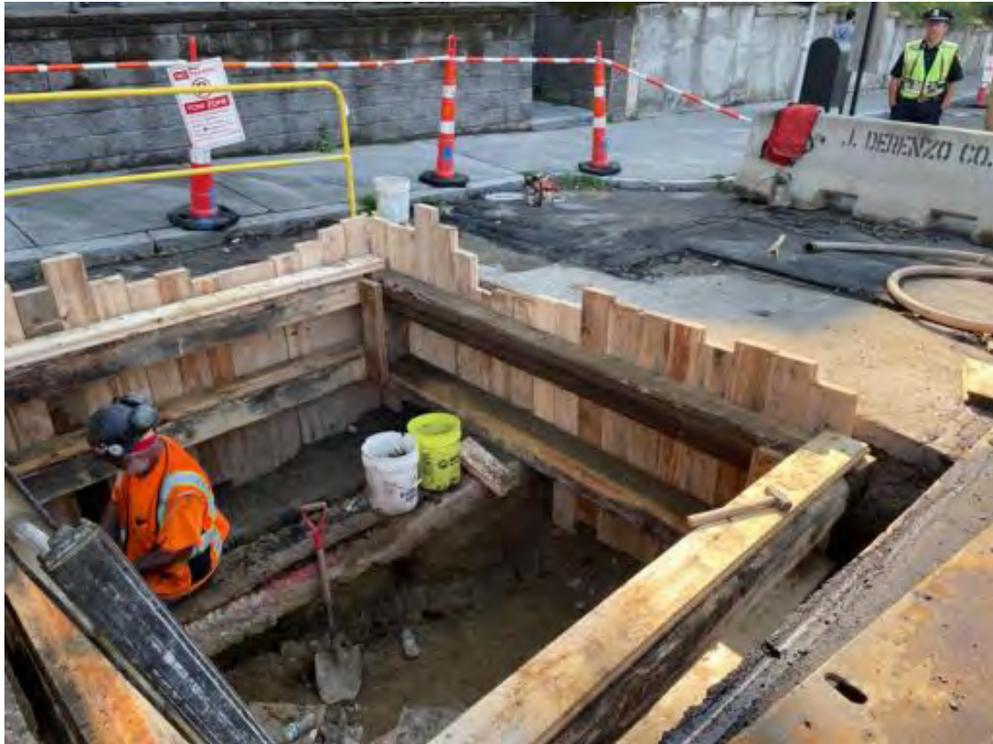
Utility work in Westbourne Terrace ongoing.
