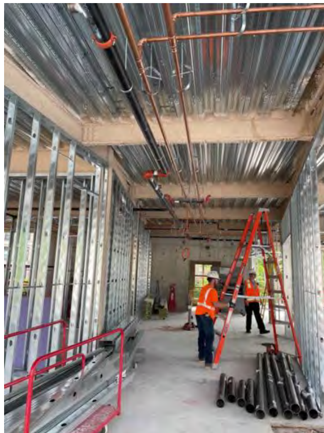
FP pipe, level 3 Area C.
