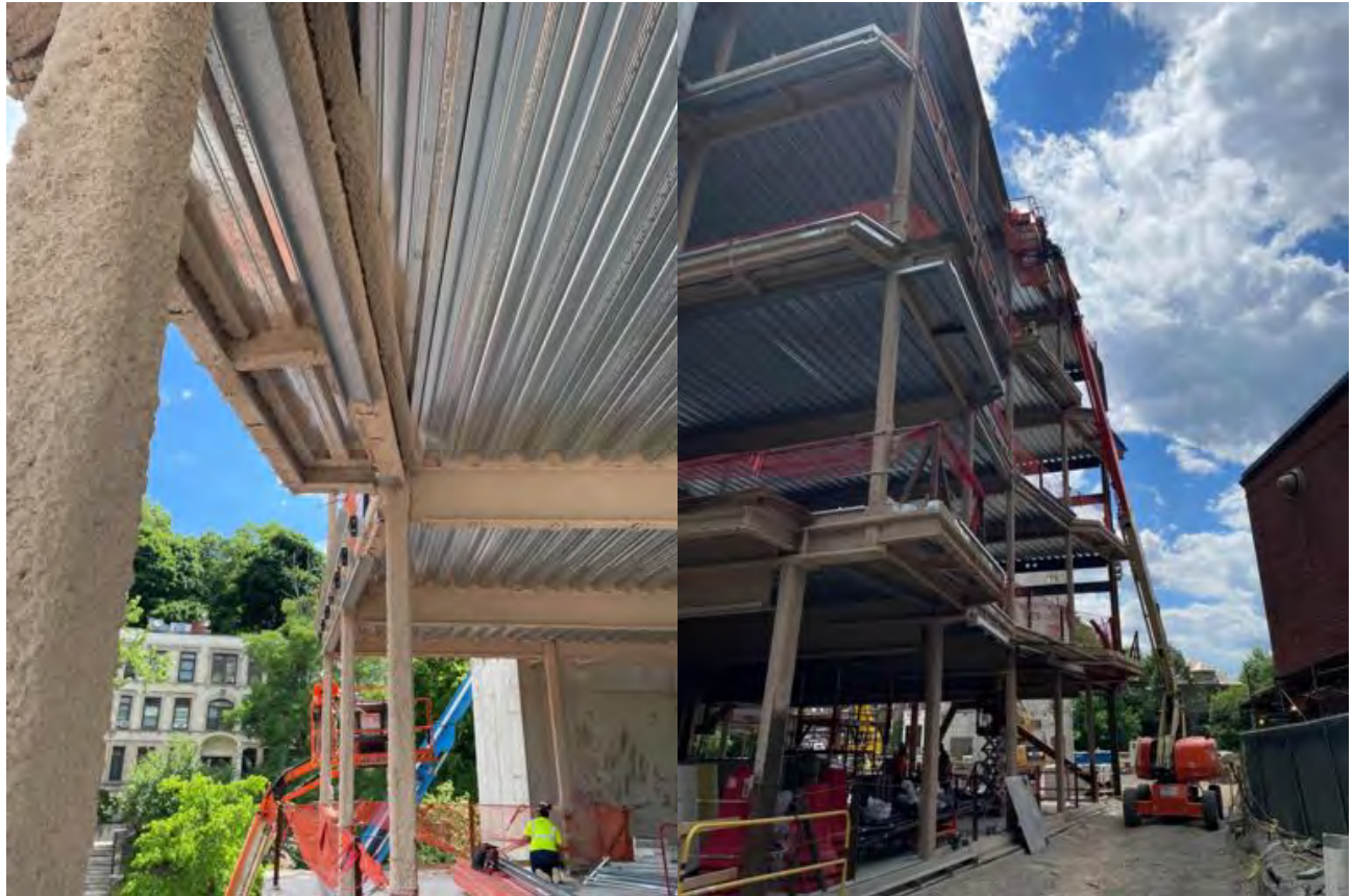
Exterior framing, West side of Area C.
