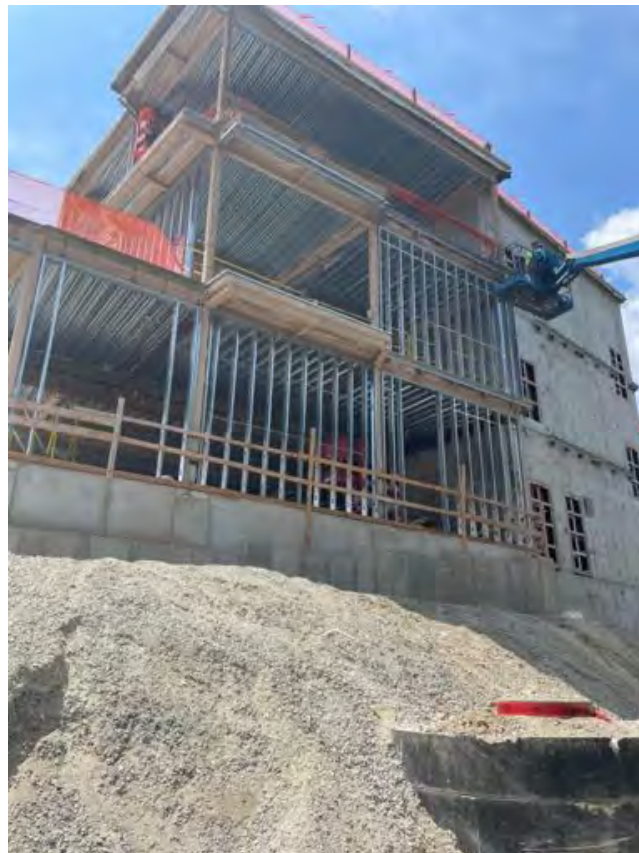
Exterior framing, North and East.
