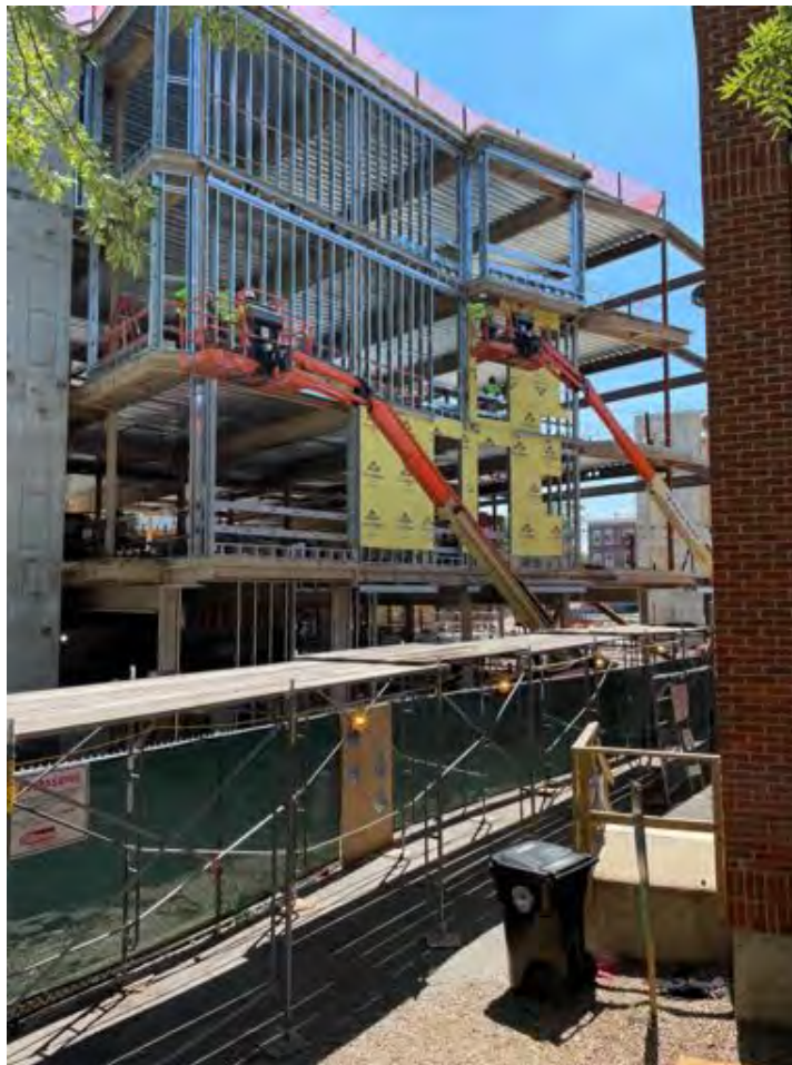
Exterior framing and sheathing, West side.
