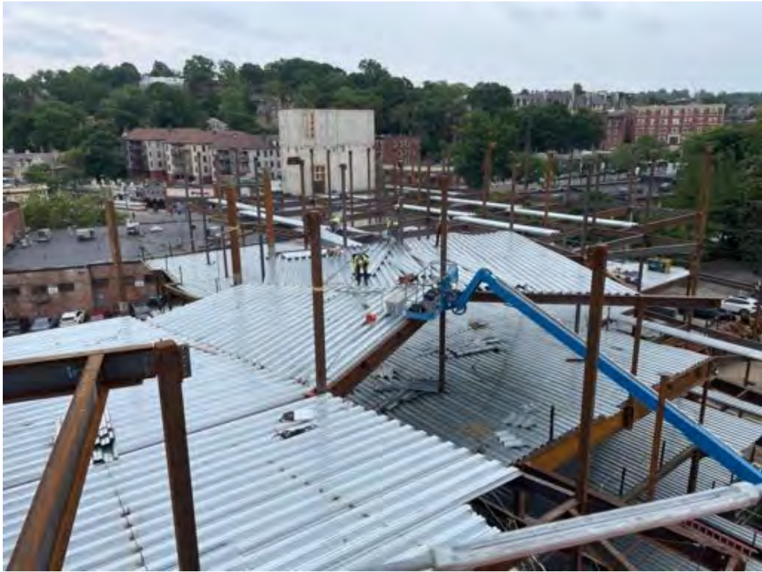
Deck installation, Level 4 Area A.
