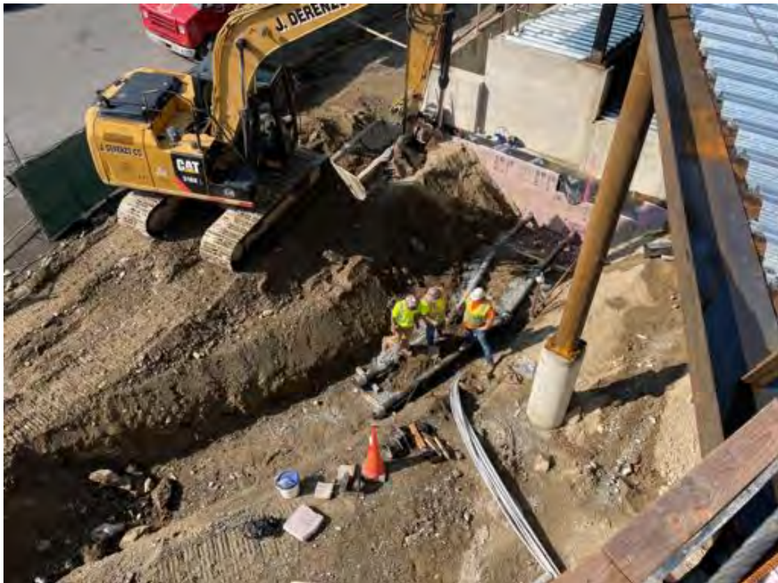
Water main exiting the building.
