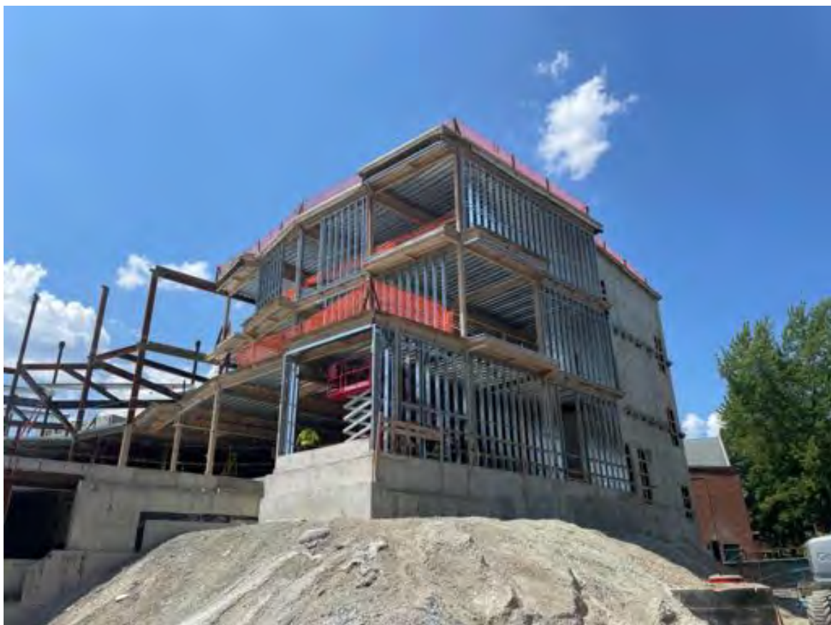
Exterior framing, North and East sides, Area C.
