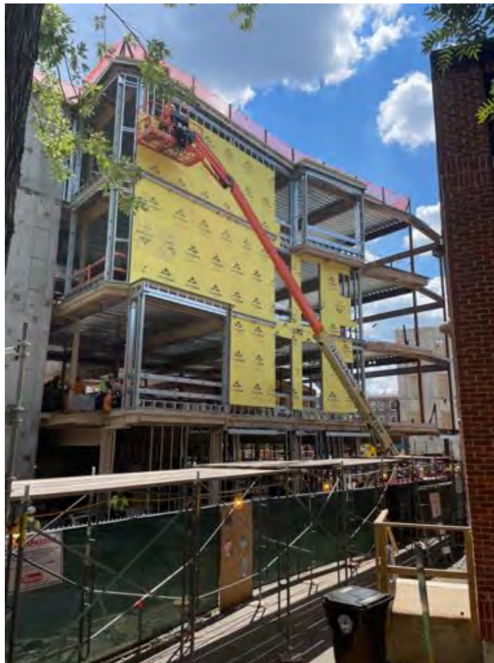
Exterior sheathing, West side.
