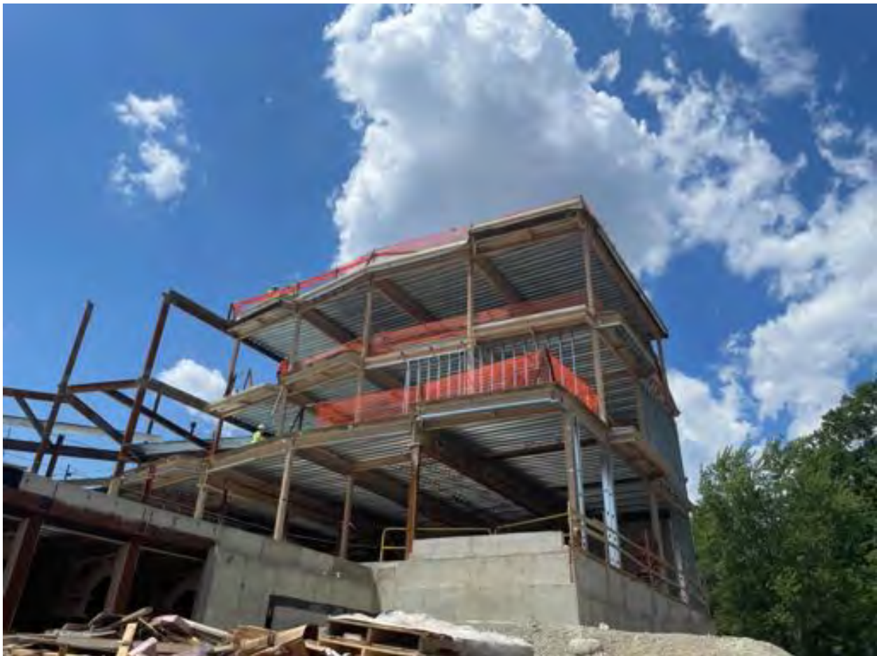
Roof blocking, Area C.
