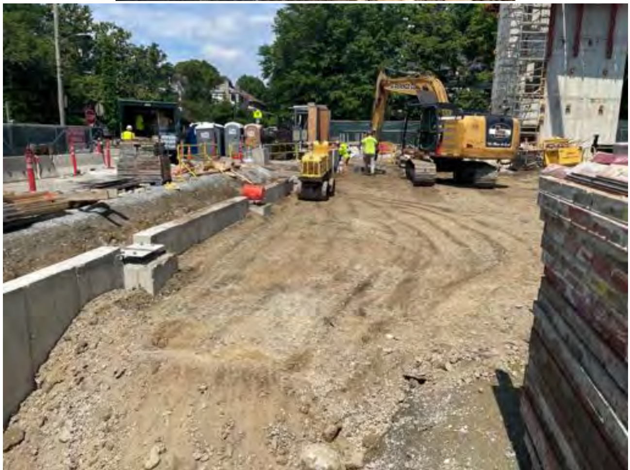
Line BD forms removed, area backfilled and compacted
