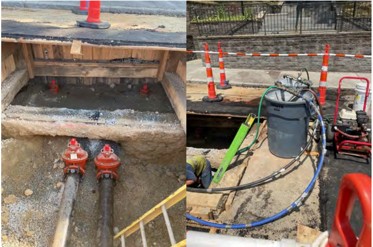
Water main and test.
