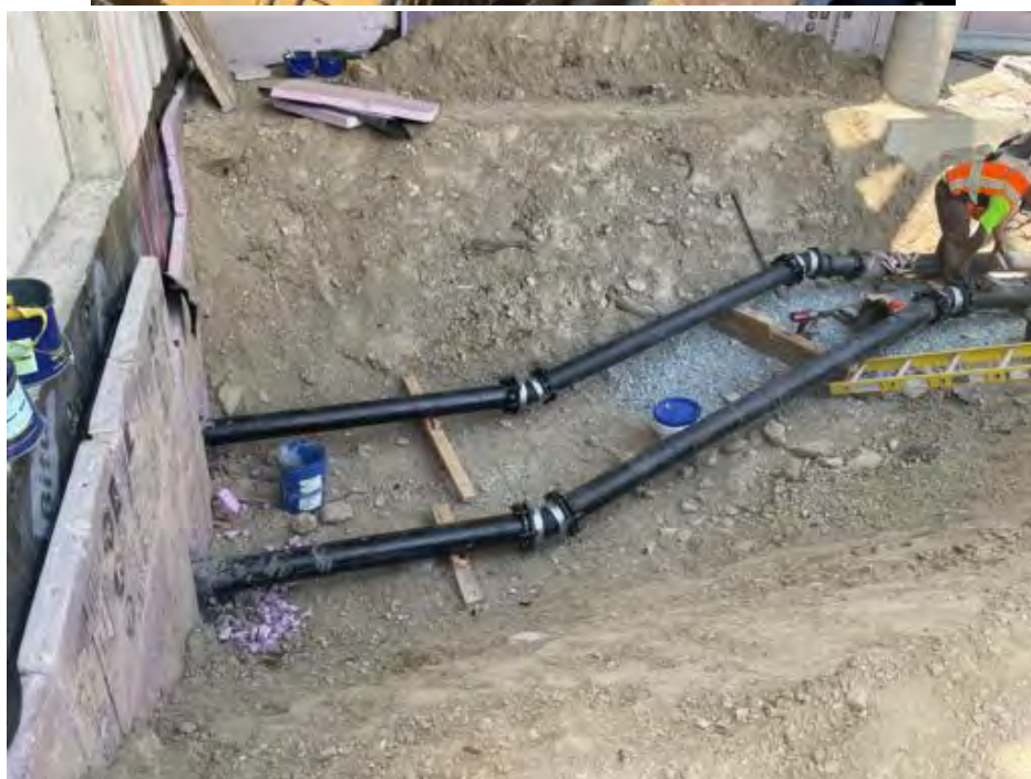
Water main exiting the building.
