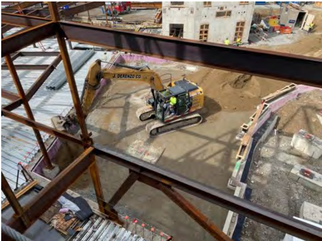
Backfill at Area A/B/C.
