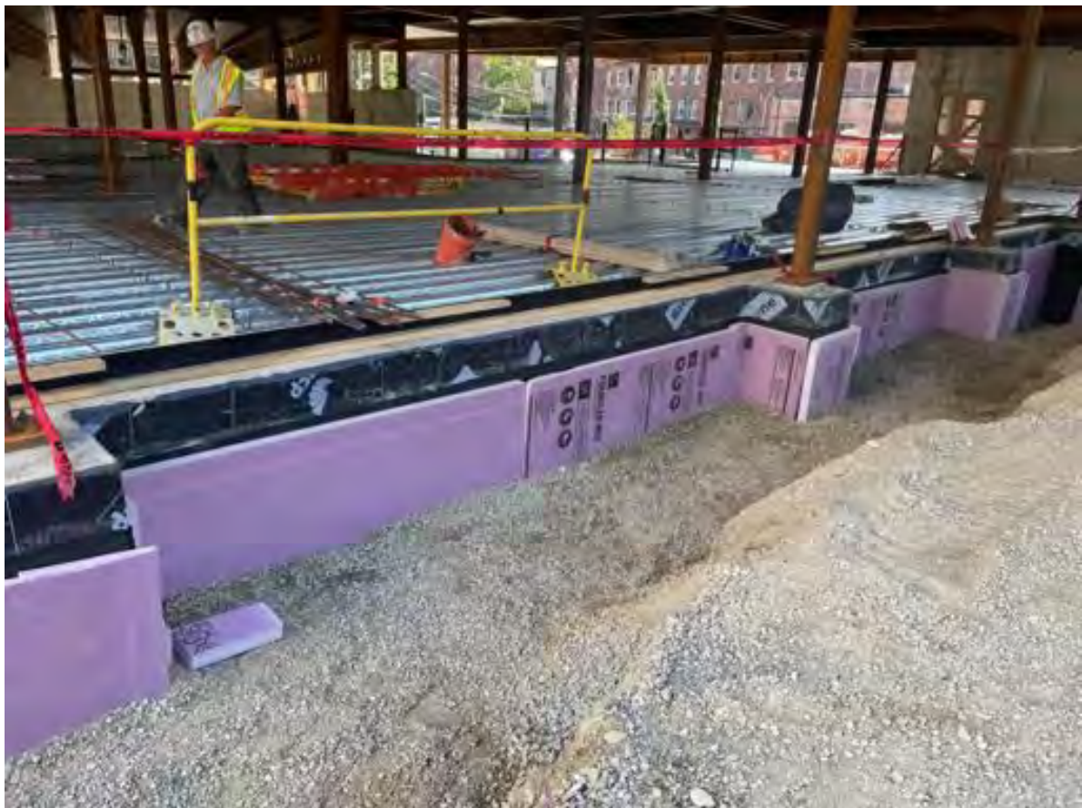
Line AG, insulated, backfilled and compacted.
