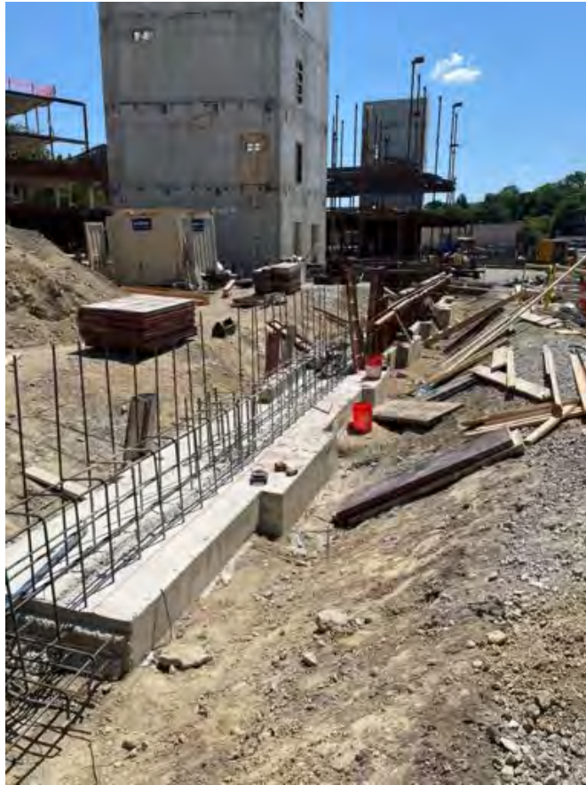
Footings at BD line stripped, wall forms started.
