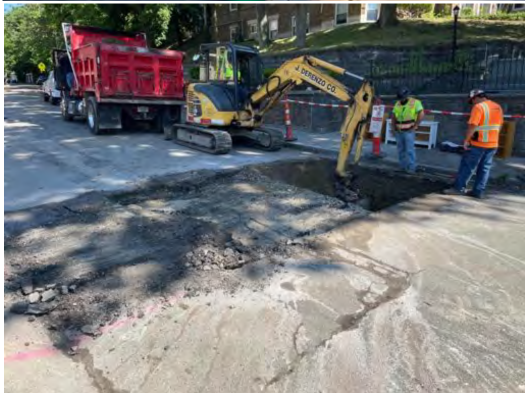
Westbourne Terrace – water connection work.
