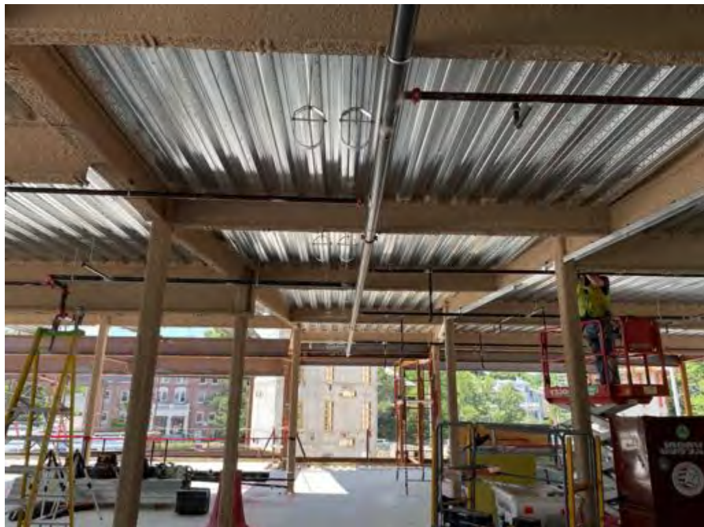
Mechanical pipe hangers installed.
