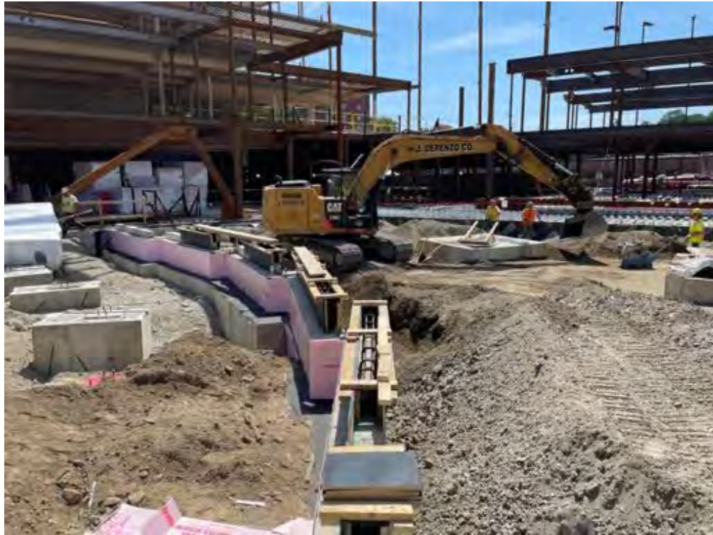
Backfill in Area A/B/C.
