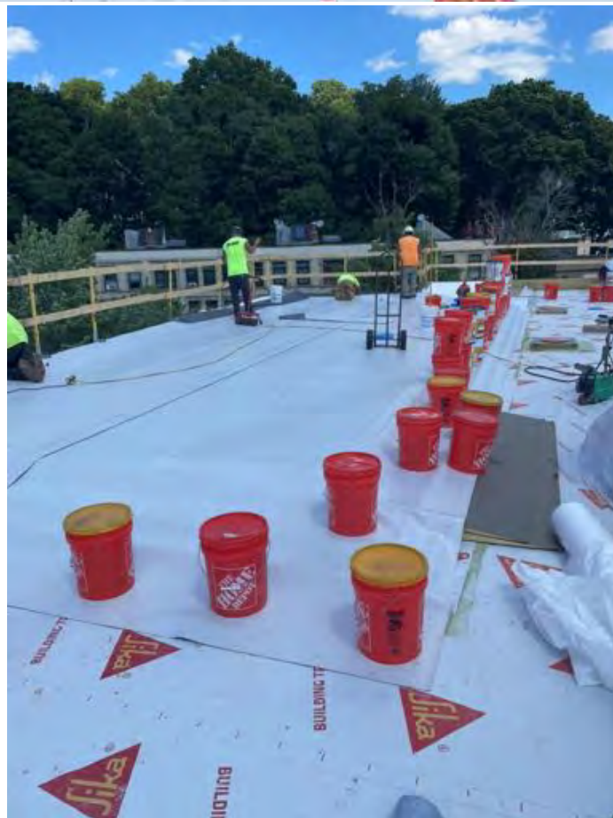
Roof progress, Area C. Insulation and membrane.
