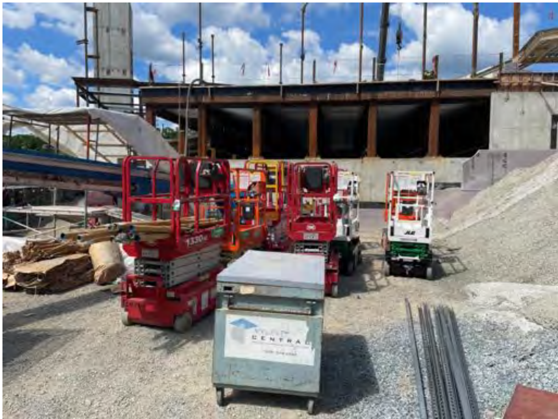
Scissor lifts delivered to site.
