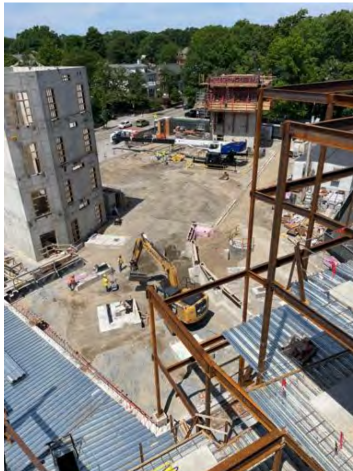
View of Area B from roof.
