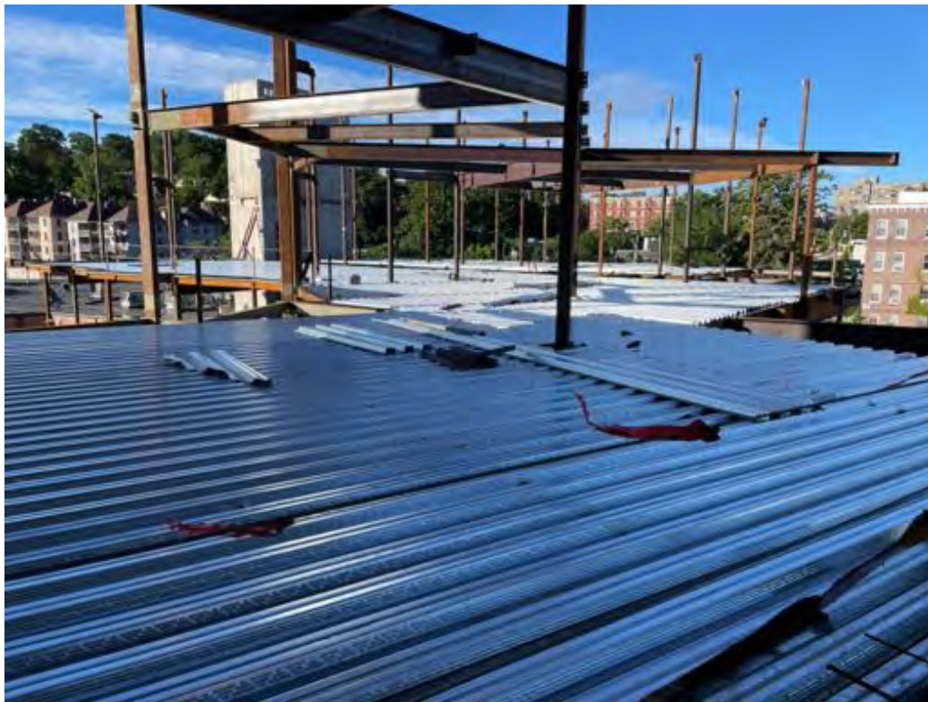
Level 3 deck installed, Area A.
