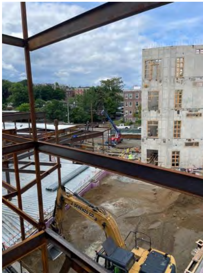
Installing steel with a lull, Area A.
