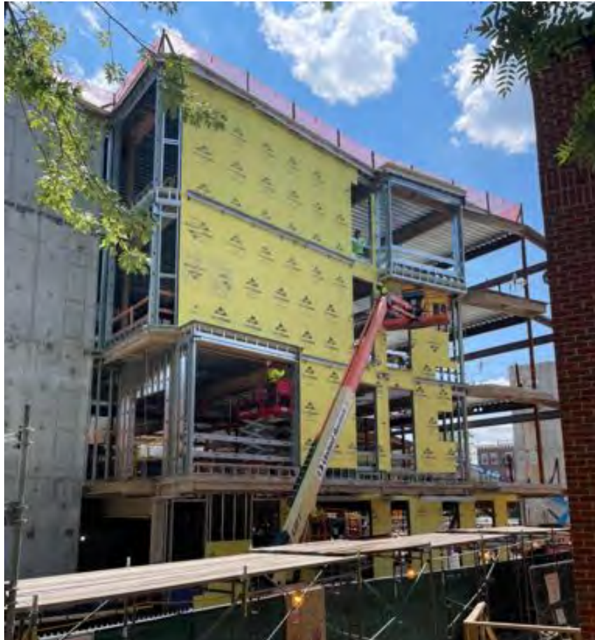
West elevation sheathing, Area C.
