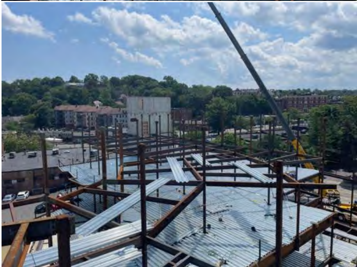
Steel erection, level 4 Area A.
