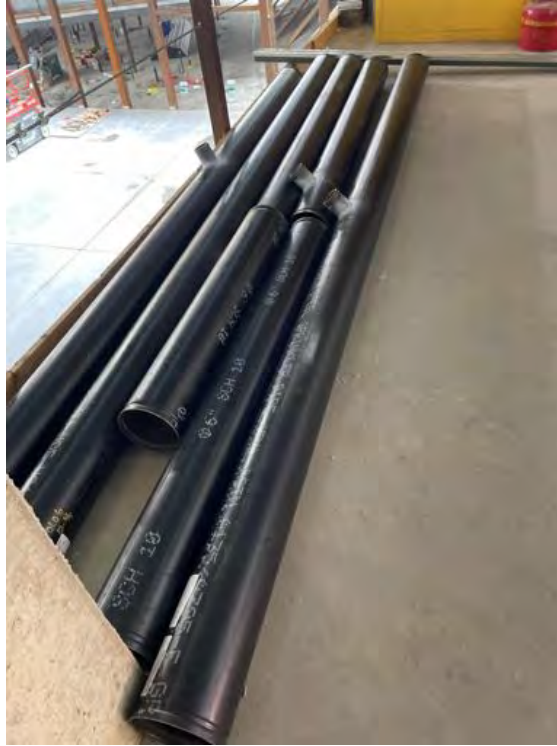
FP pipe staged.
