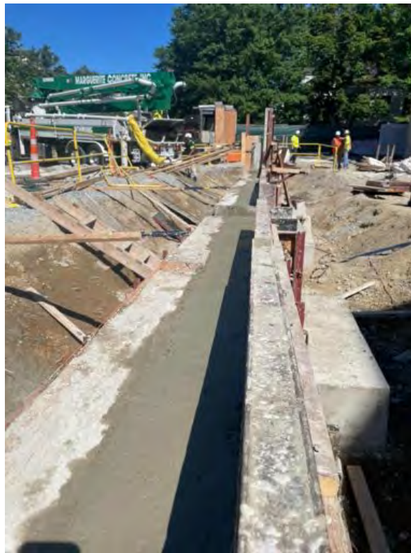
Concrete foundation wall at line BD poured.
