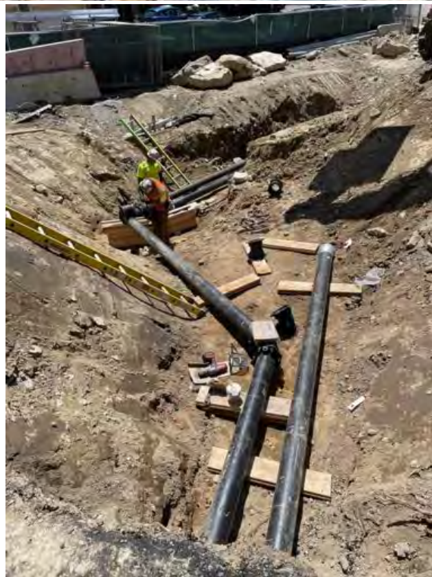
Water main work.
