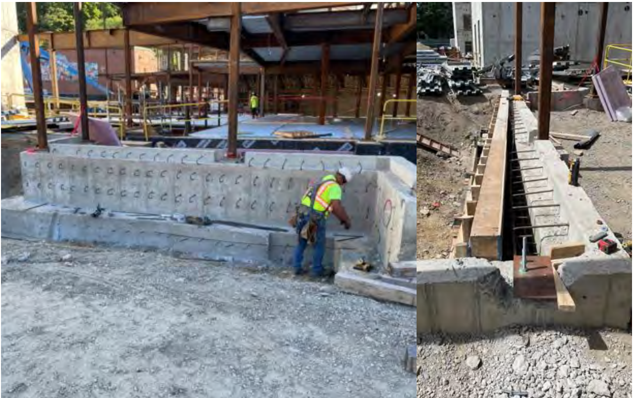
Rebar for foundation repair, line AD.
