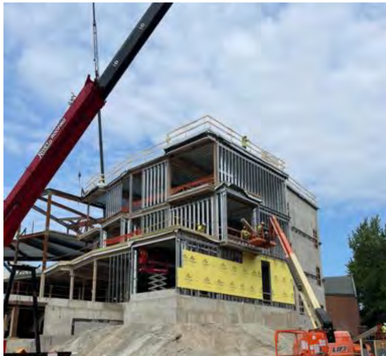
Northeast elevation, Area C.
