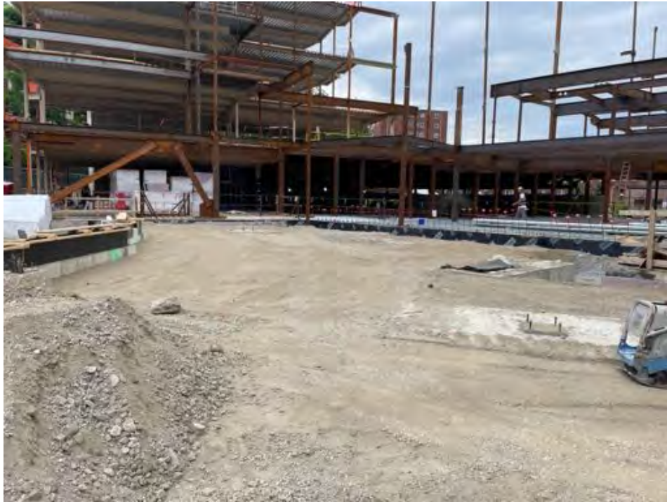
Compaction at Area A/B/C.
