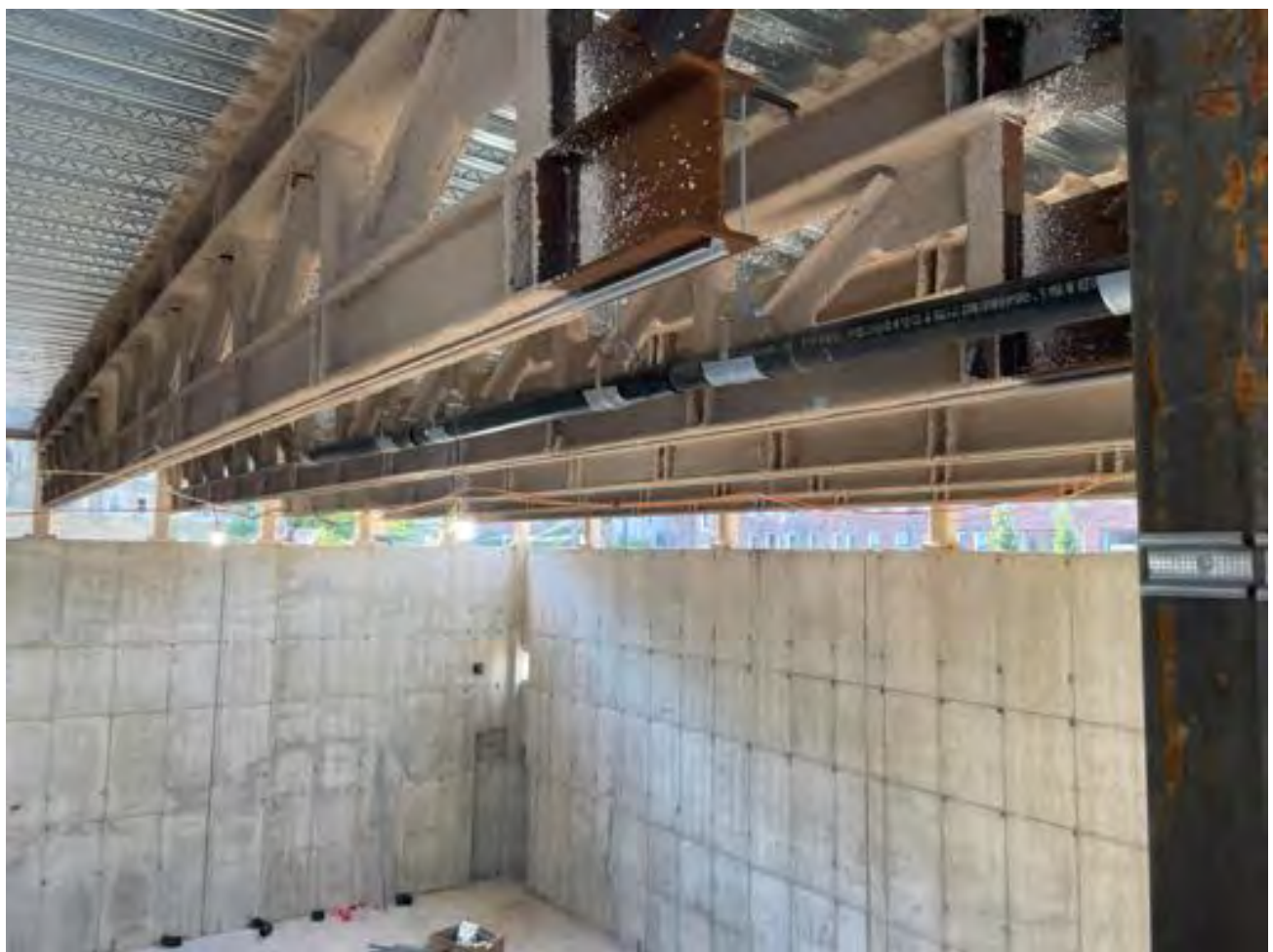
Plumbing above gym.
