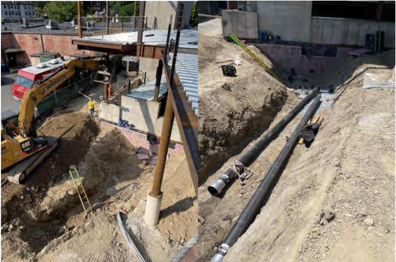
Water main excavation/installation.
