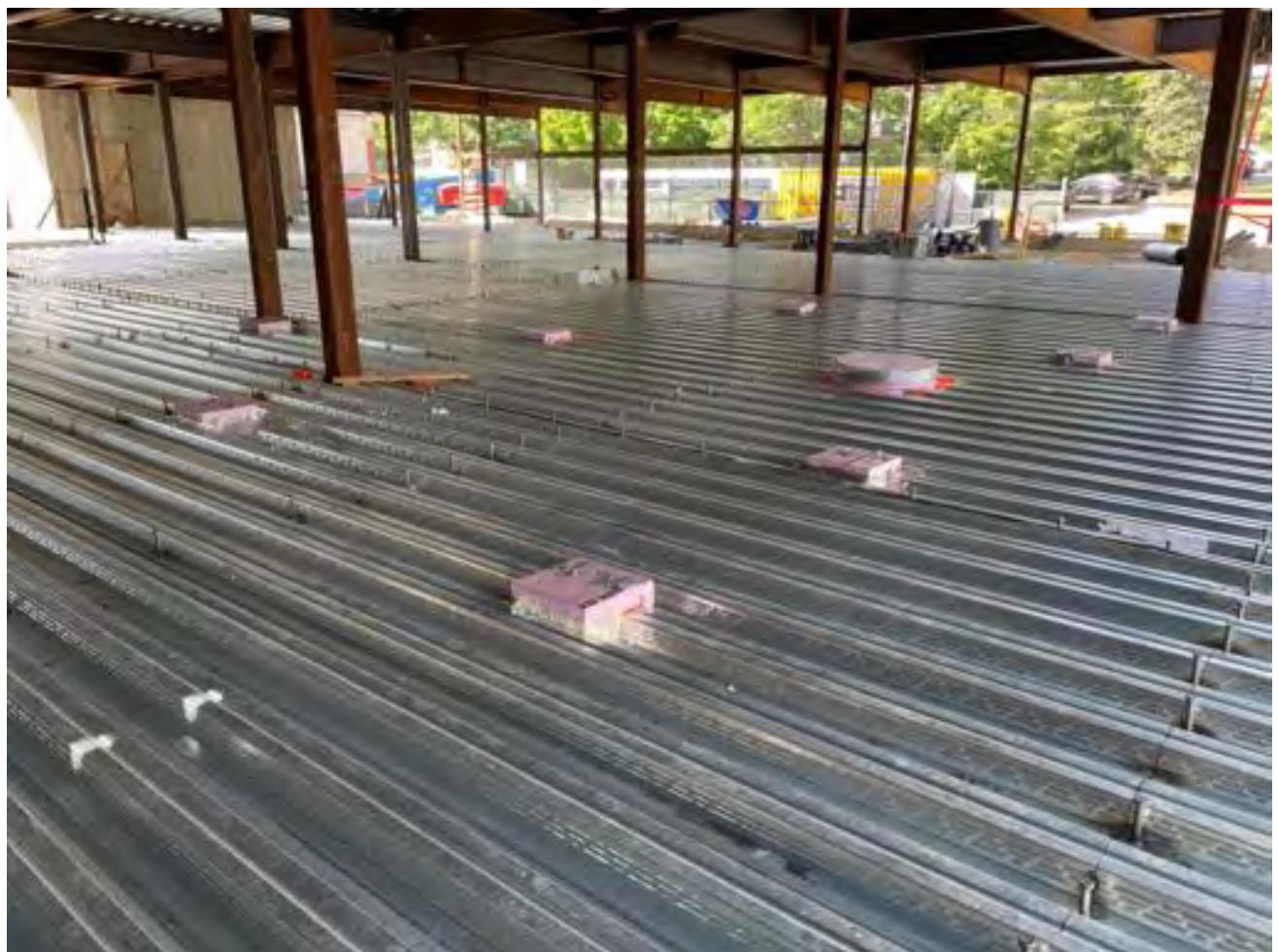
Plumbing blockouts, Area A.
