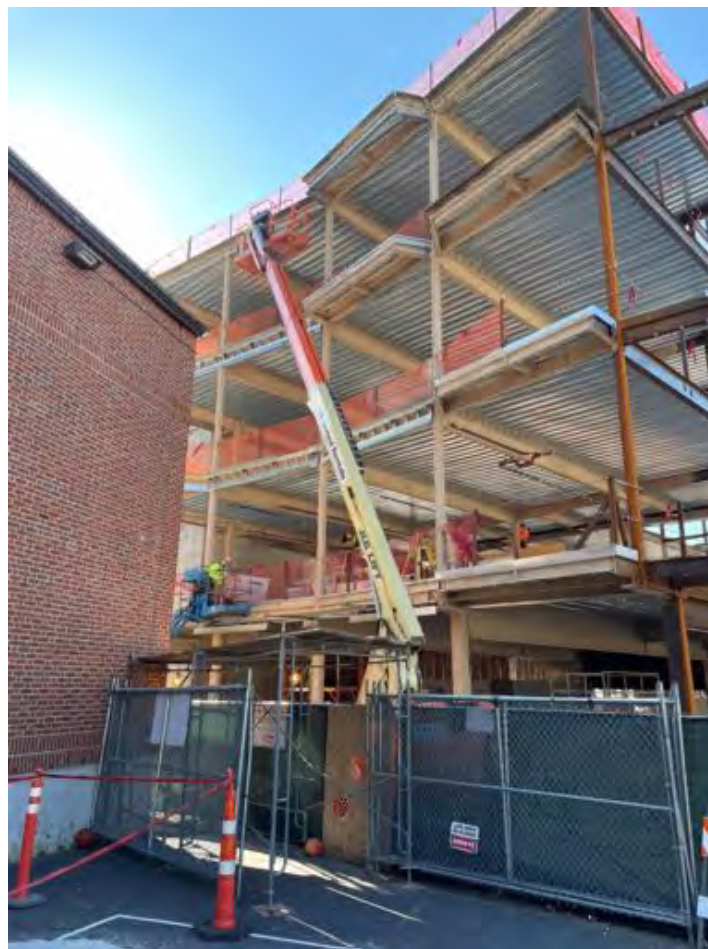
Exterior framing, West side.
