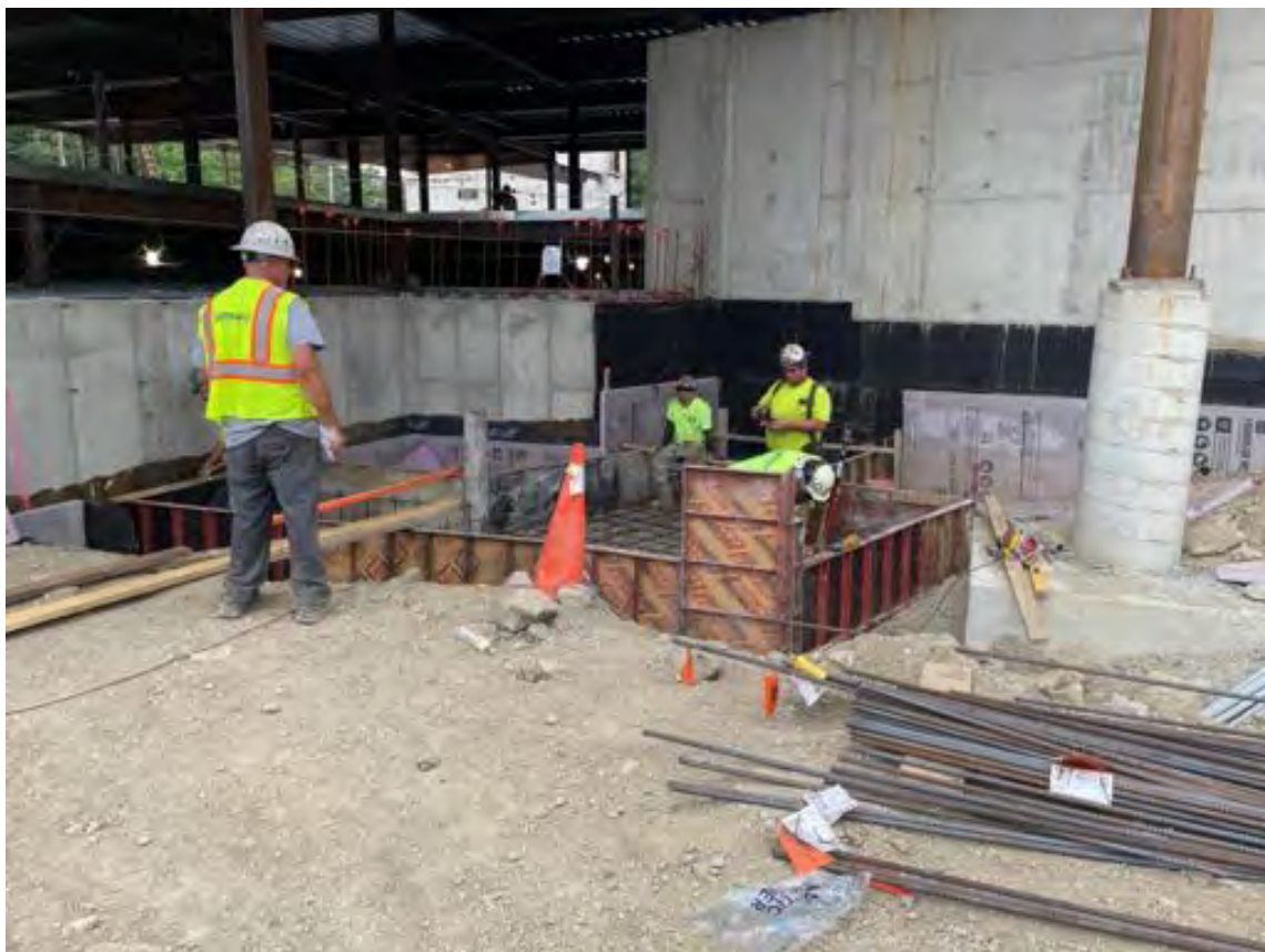
Loading dock slab – forms and rebar.
