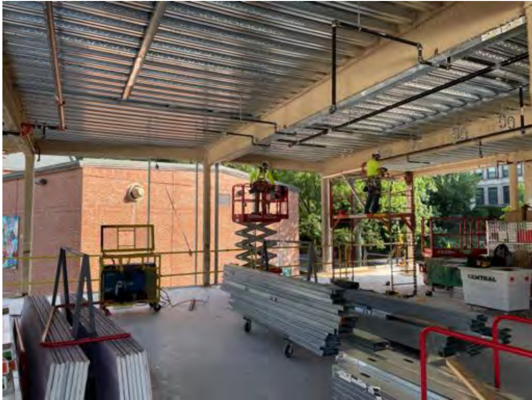
Hangers and framing, second floor Area C.
