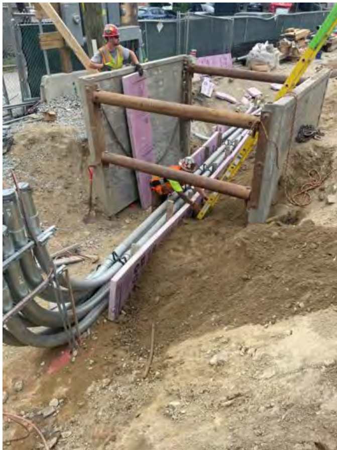
Electrical ductbank at transformer pad location.
