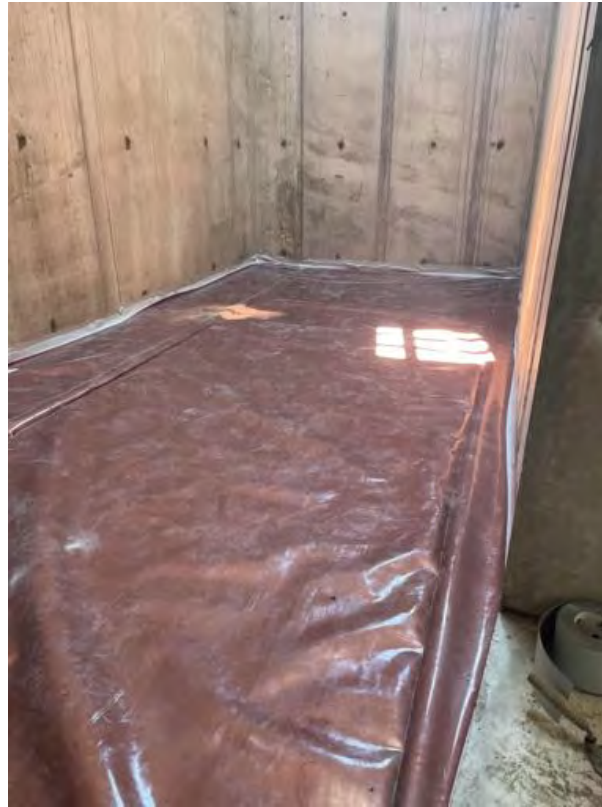
Bottom of Core A, ready for concrete.
