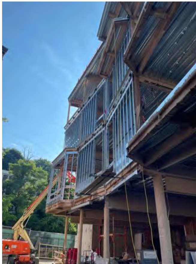
Exterior framing, West side.
