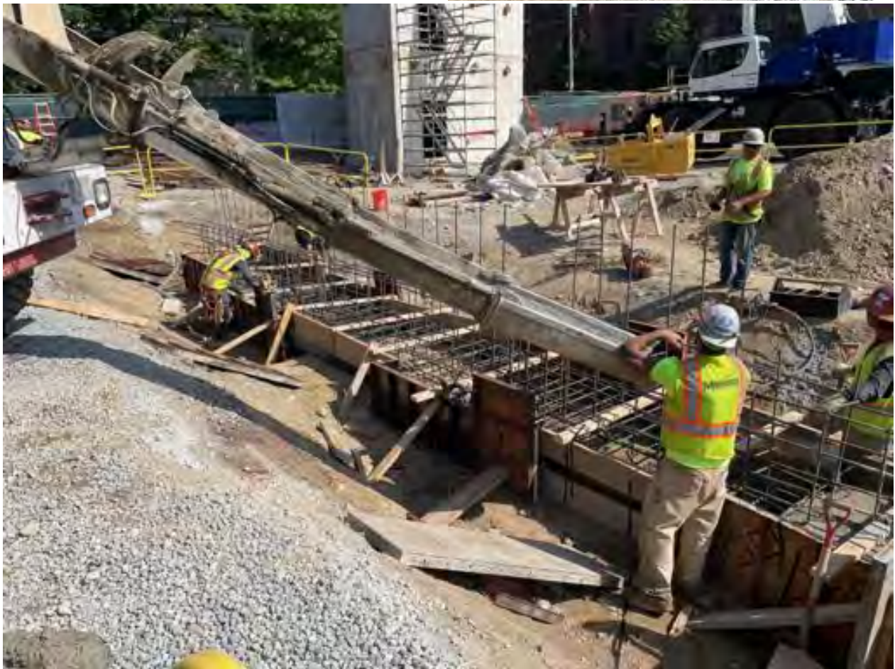
Footings at line BD, South.
