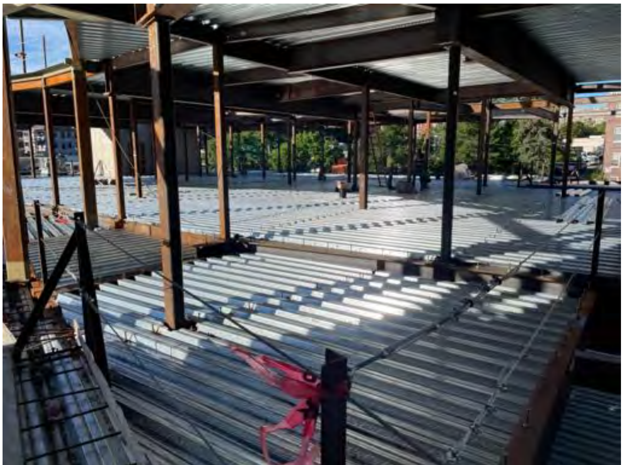
Deck studs welded, levels 1 and 2.
