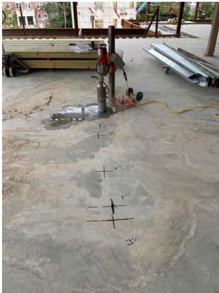
Prep for plumbing cores.
