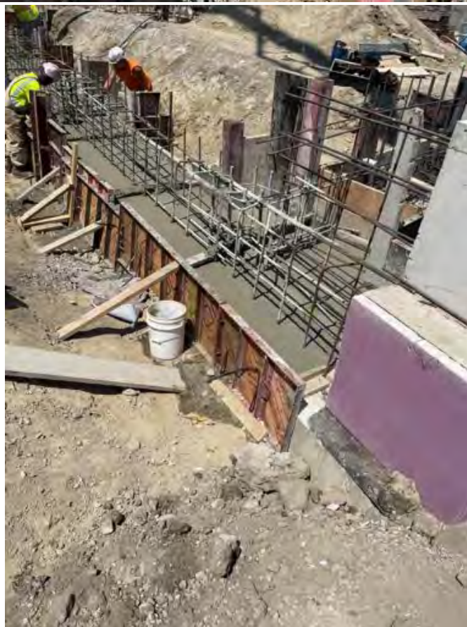
Forms, rebar and concrete, Area B.
