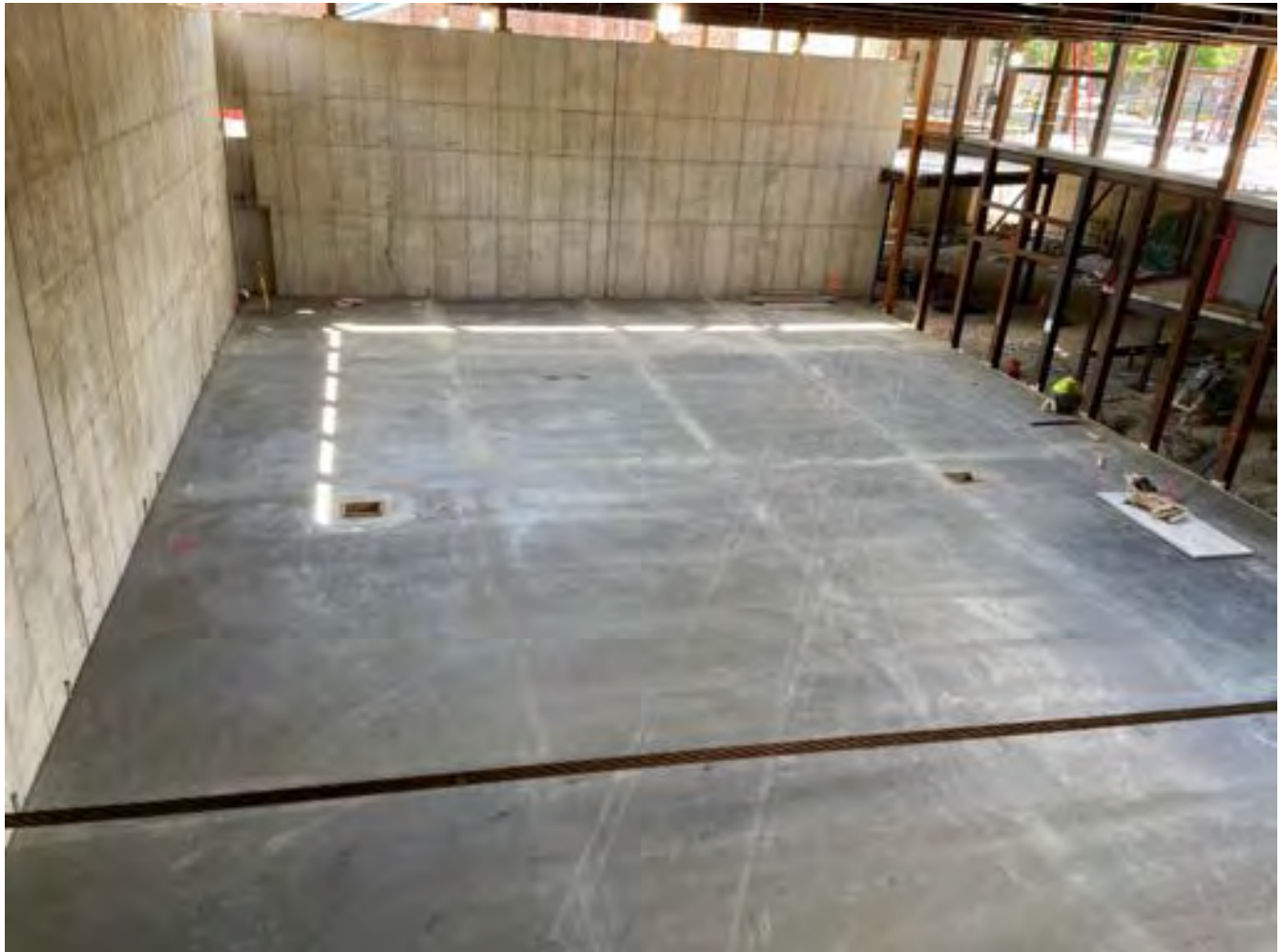
Gym slab on grade.
