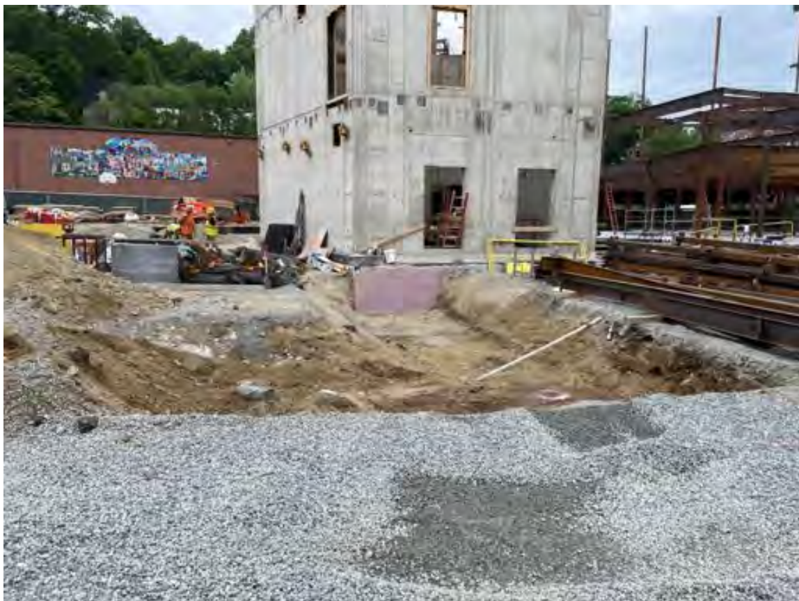
Excavation for footings, Area B.
