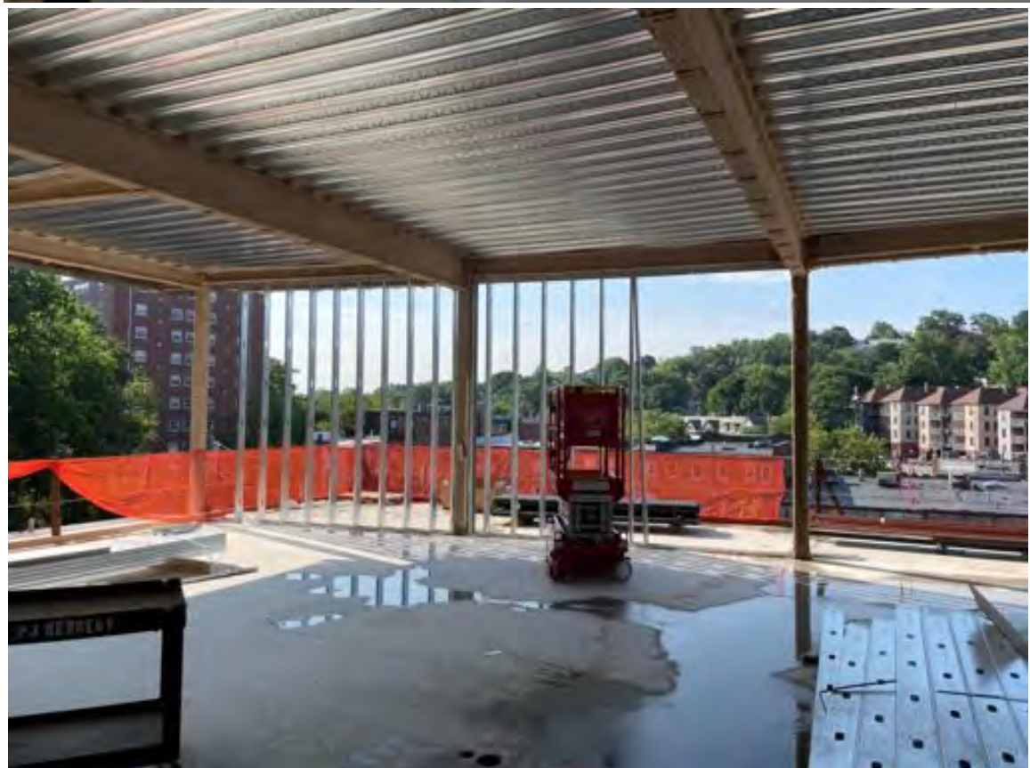
Exterior framing, East and West 3 rd floor.
