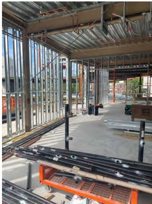
Level 3 exterior framing.
