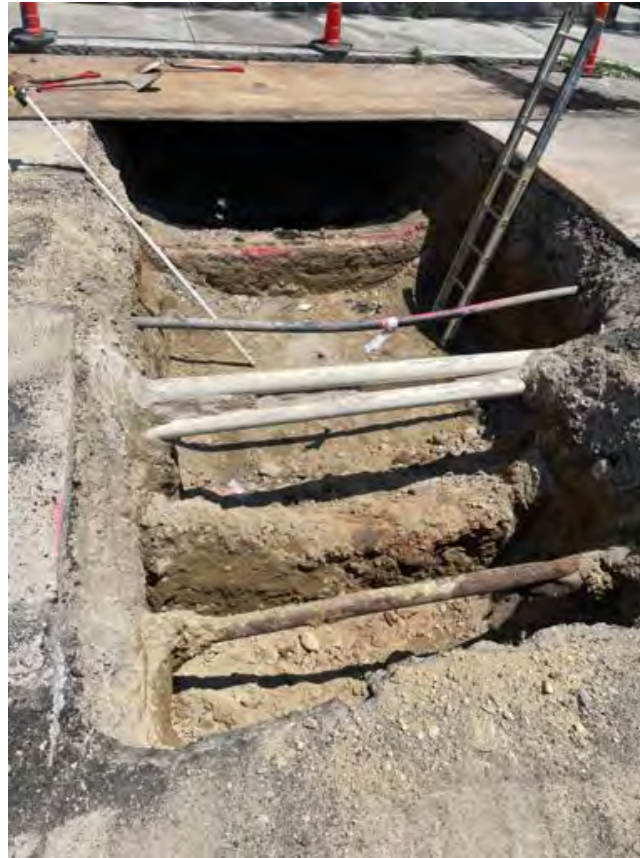
Westbourne Terrace work ongoing, utilities exposed.
