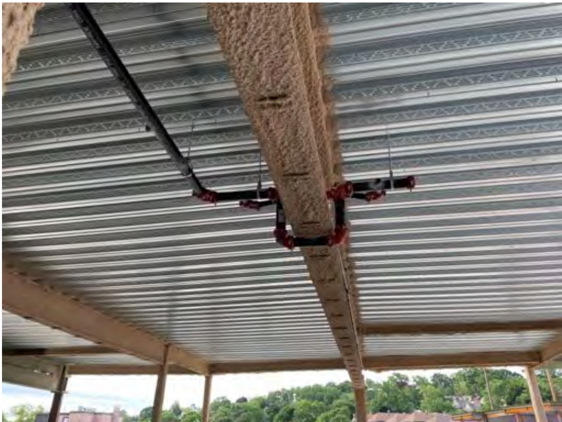
Fire protection pipe, level 2 Area C.
