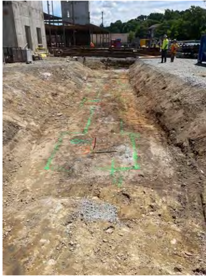
Excavation for footings, Area B south.
