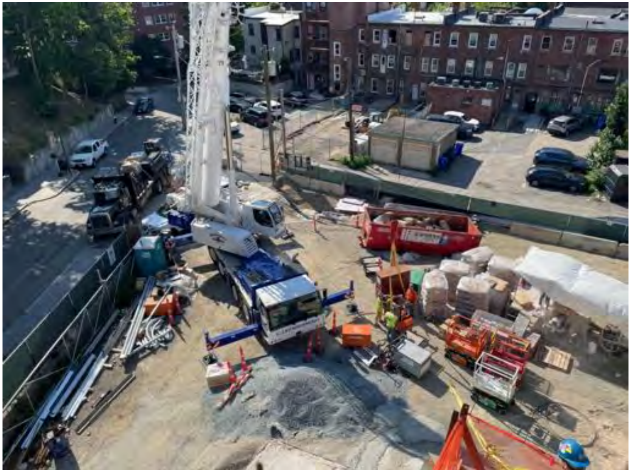
Crane pick of materials and equipment.
