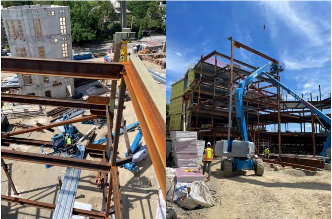
Steel erection, Area C/A.
