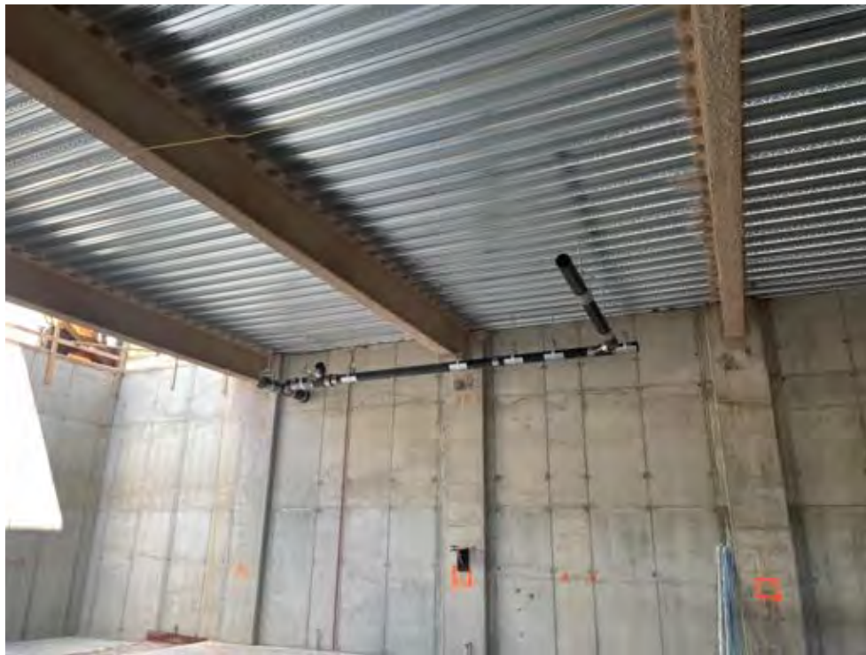
Storm pipe, small gym.
