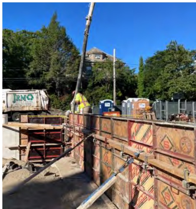
Concrete pour, line BD foundation.
