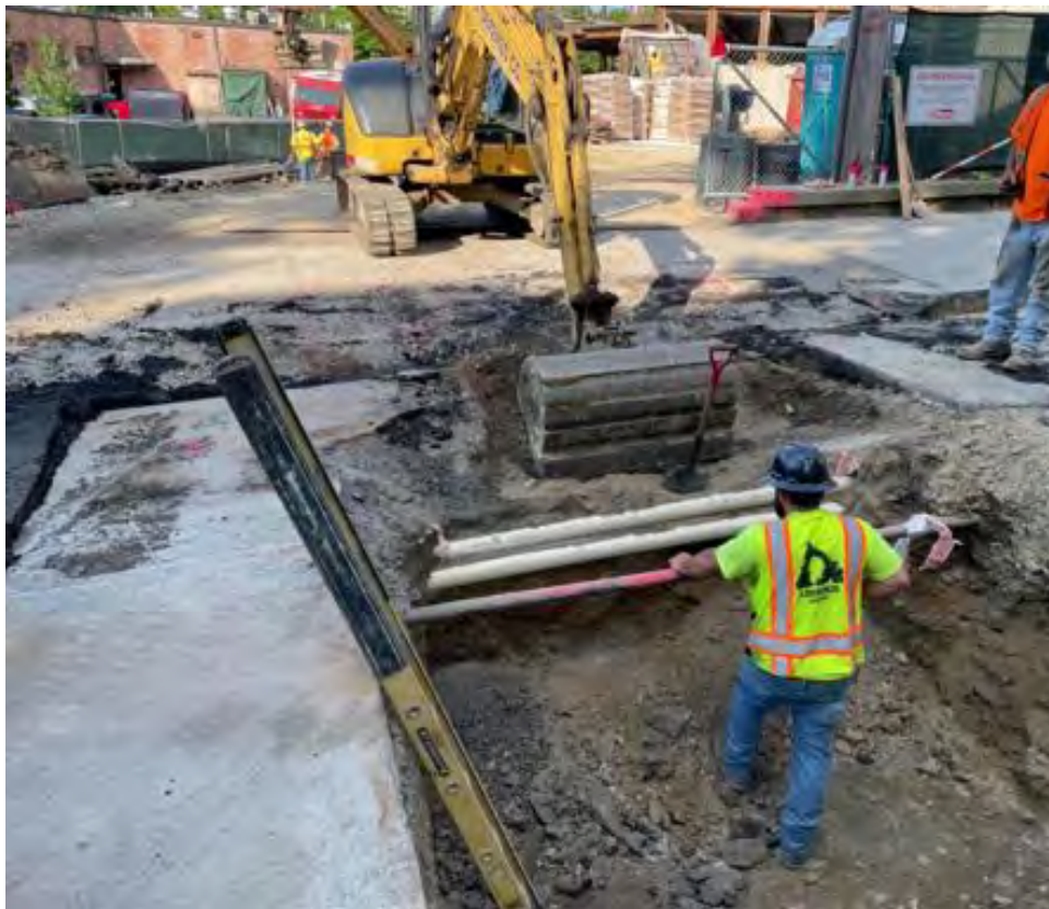
Westbourne Terrace water connection ongoing. No surprises.
