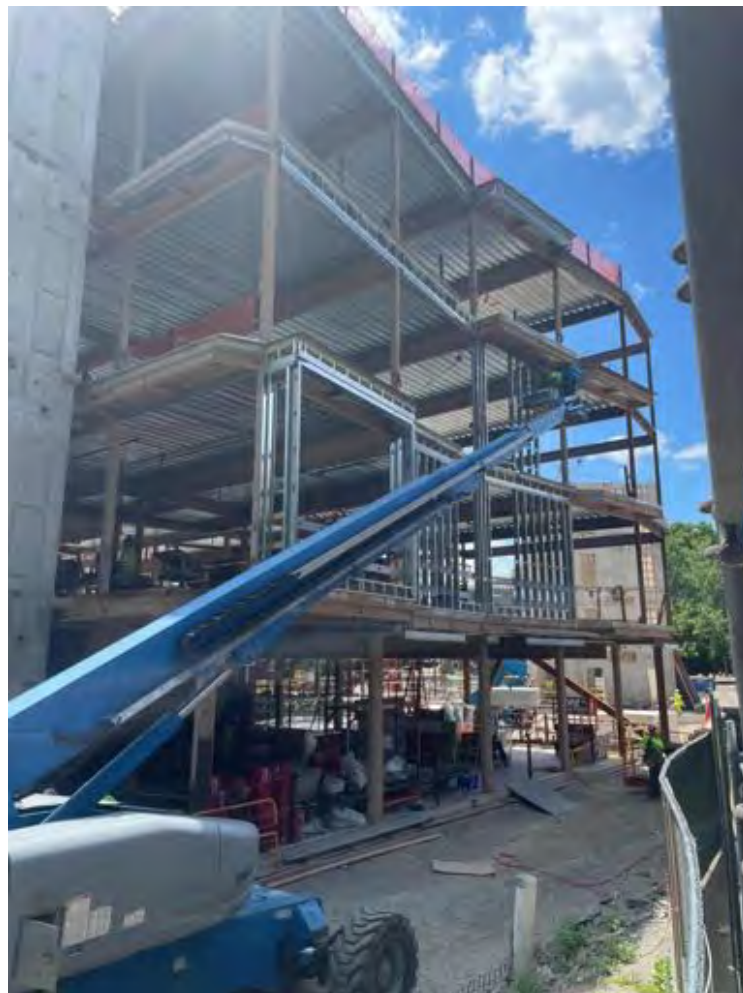
Exterior framing, West wall.
