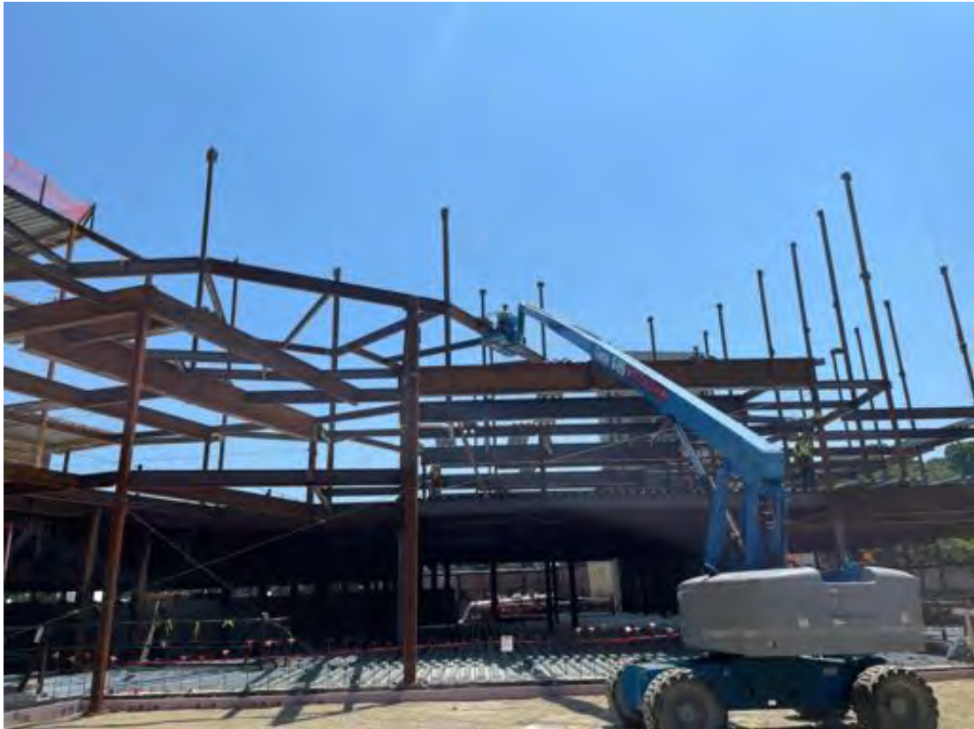
Steel erection ongoing.
