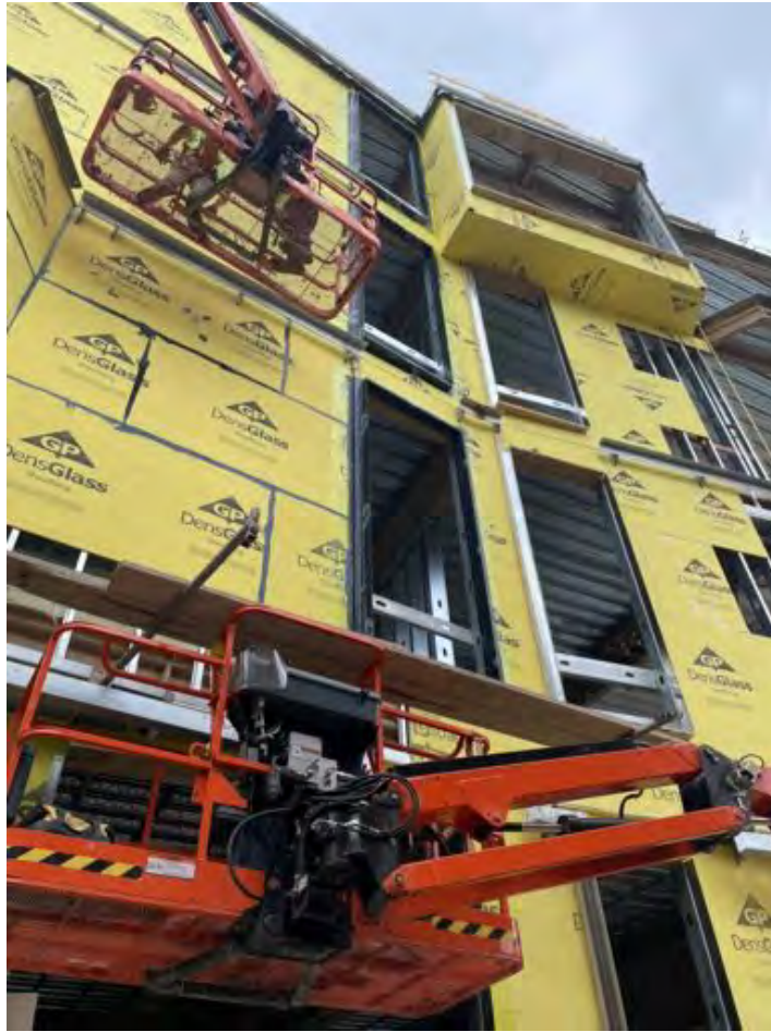
Waterproofing, West elevation Area C.
