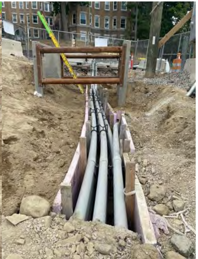
Electrical ductbank at transformer pad location.
