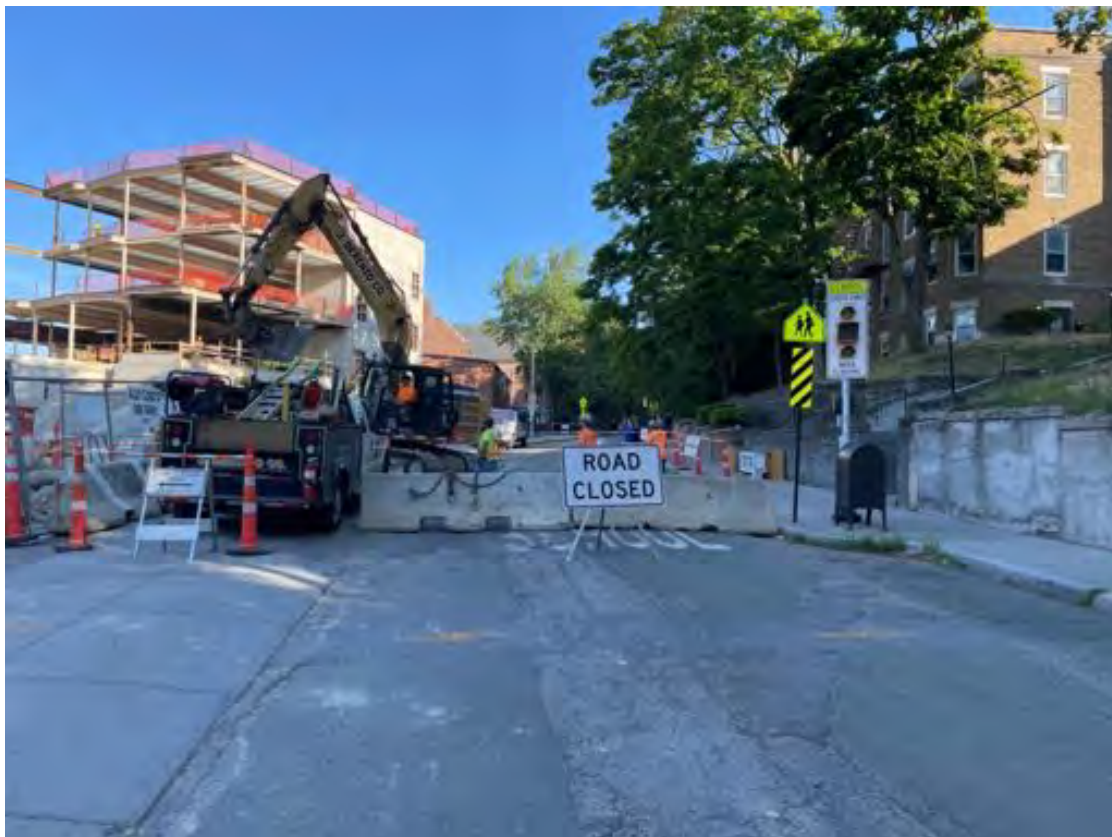
Westbourne Terrace closed for water connection work.
