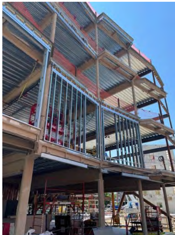
Exterior framing, West side.
