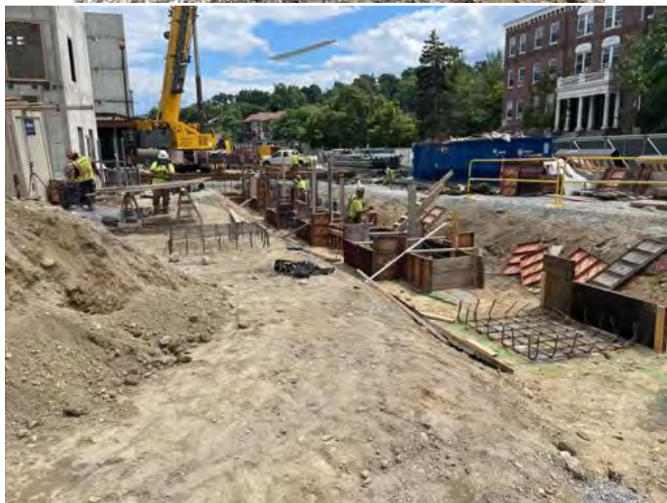
Excavation, forms and rebar for footings, South side of Area B.
