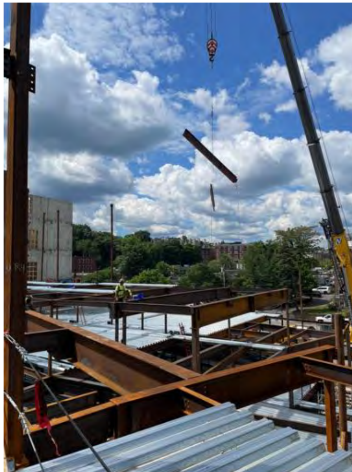
Steel erection, Area A.
