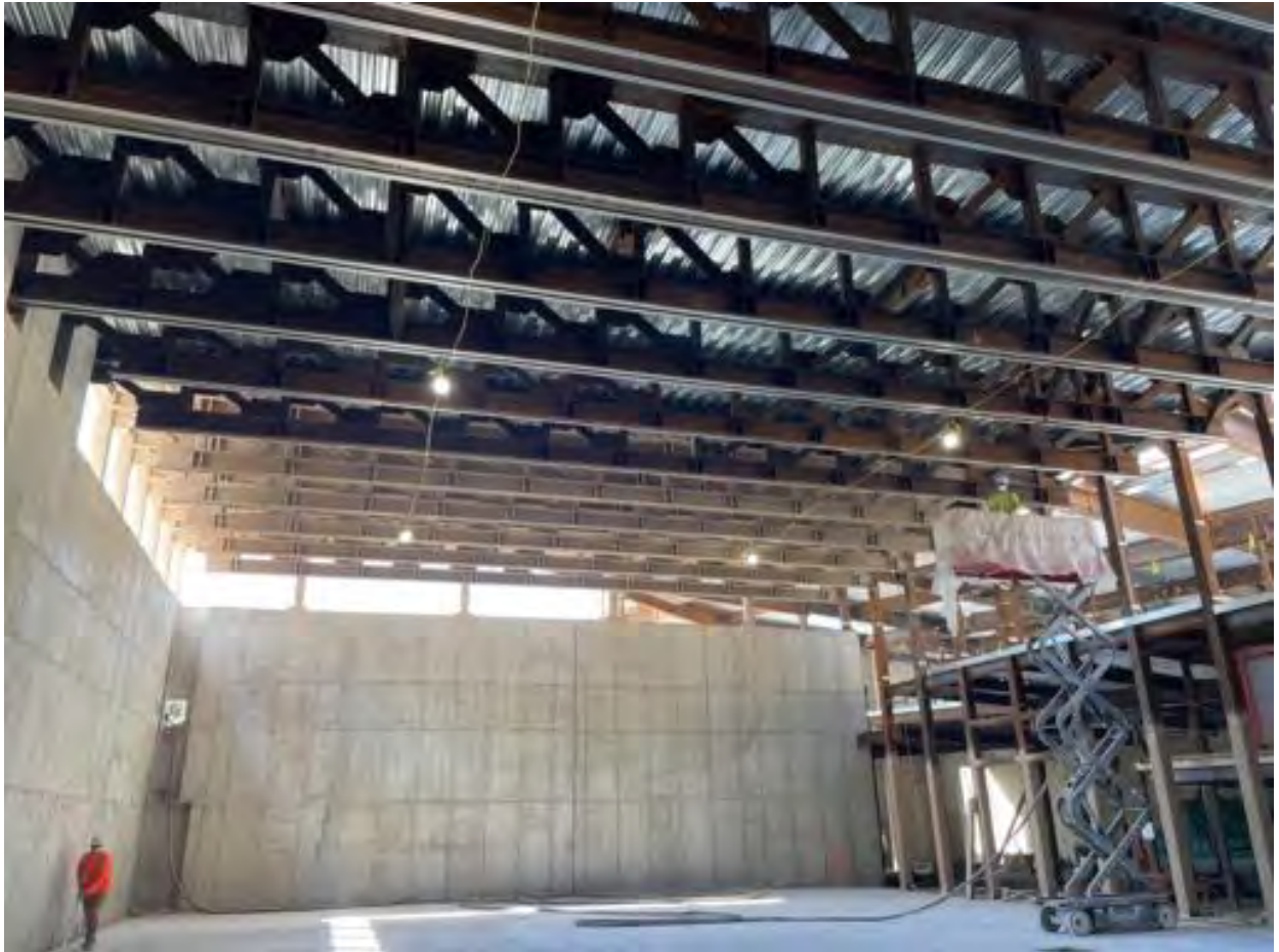
Spray-on fireproofing, gym trusses.
