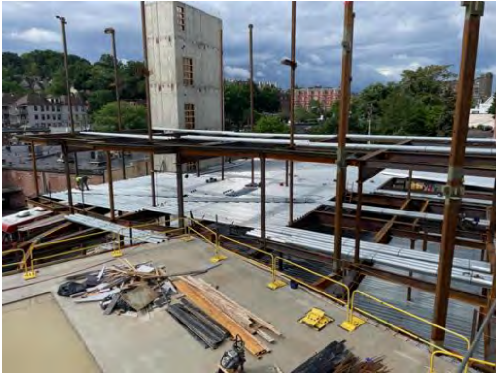
Decking, Level 2 Area A.
