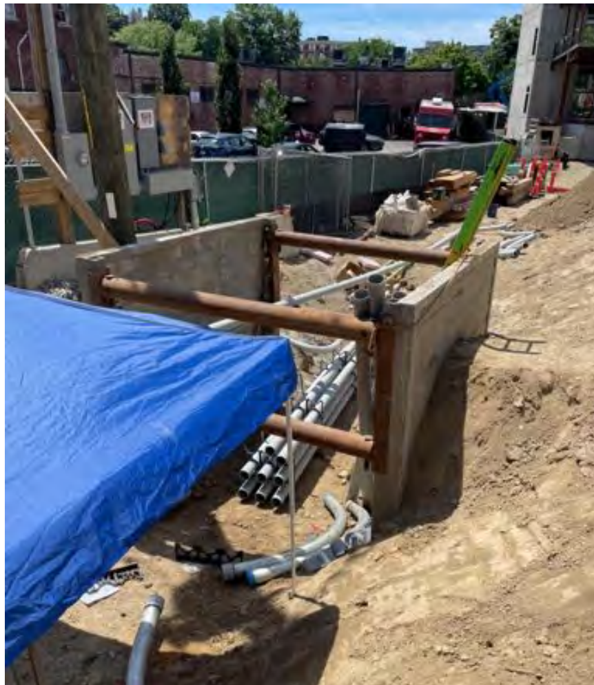
Electrical ductbank work ongoing.
