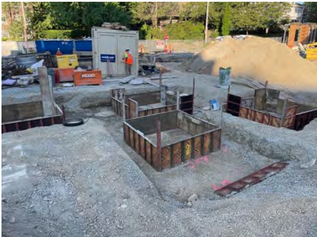
Footings in Area B ready for concrete.
